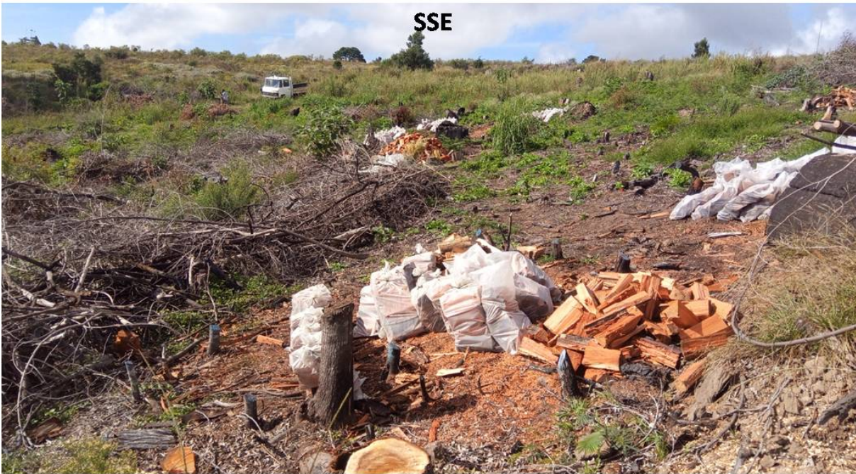
Figure 18. Tree felling and wood cutting operations on slopes of drainage line in the north-eastern quadrant of RE/21/195.
