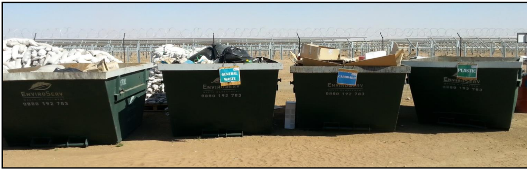
Image 1: Recycling system implemented on a construction site. Skips provided for general waste, plastic, cardboard and metal.
