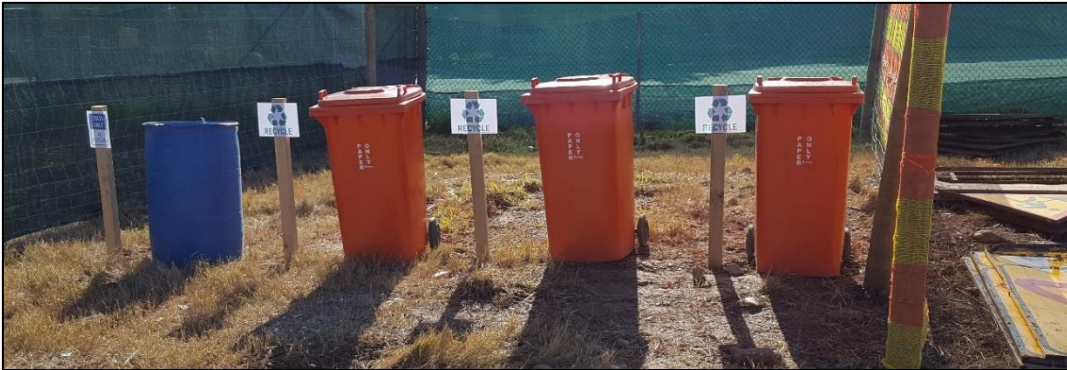
Image 2: Recycling system implemented on a construction site. Lidded bins provided for general waste, plastic, cardboard, and metal.
