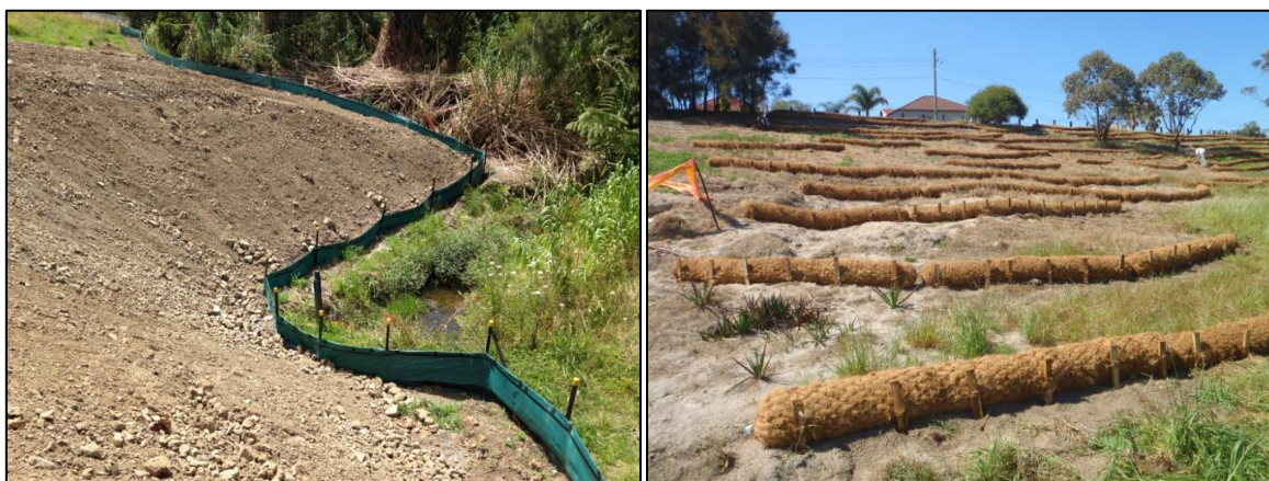
Figure 12: Examples of silt fences (left) and coir logs (right) used to trap sediment mobilised from steep slopes.
