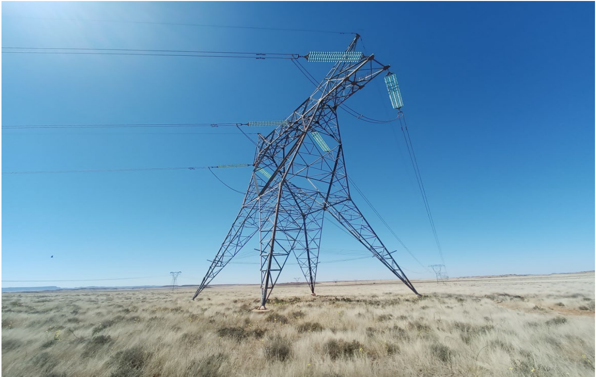
Figure 59: scale of infrastructure
