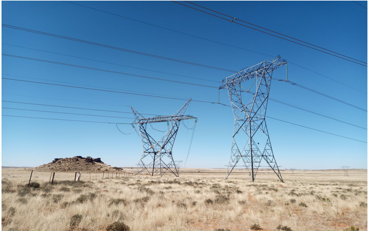
Figure 55: pylons in foreground, koppies in middle distance
