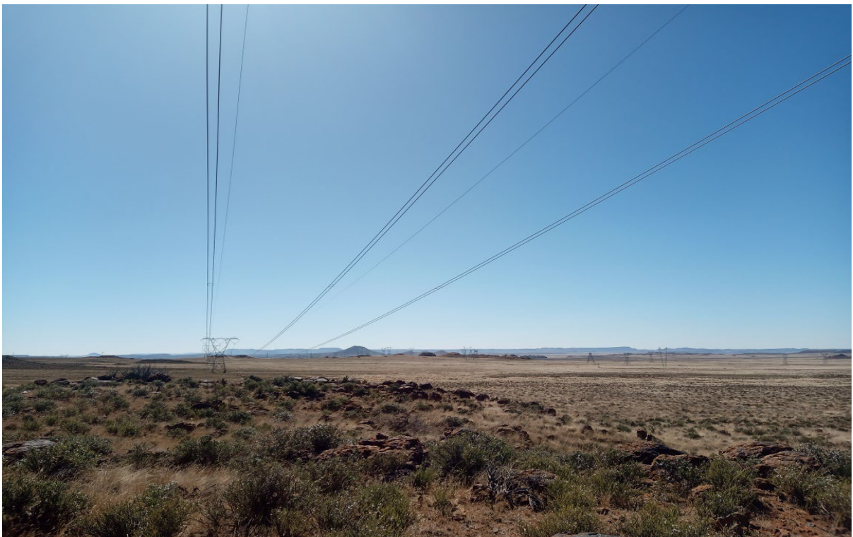
Figure 48: dolerite ridge with existing gridline
