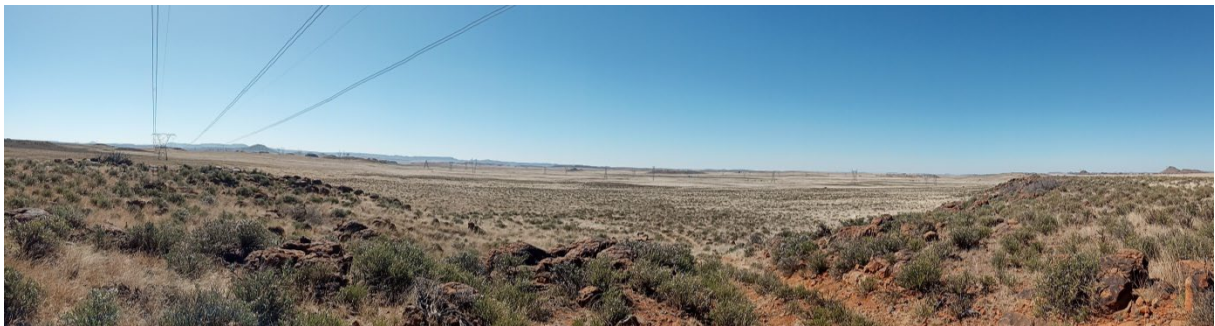
Figure 25: panoramic view from ridgeline towards existing powerlines
