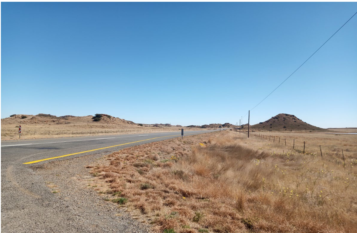
Figure 38: N10 extending northwards from the site entrance
