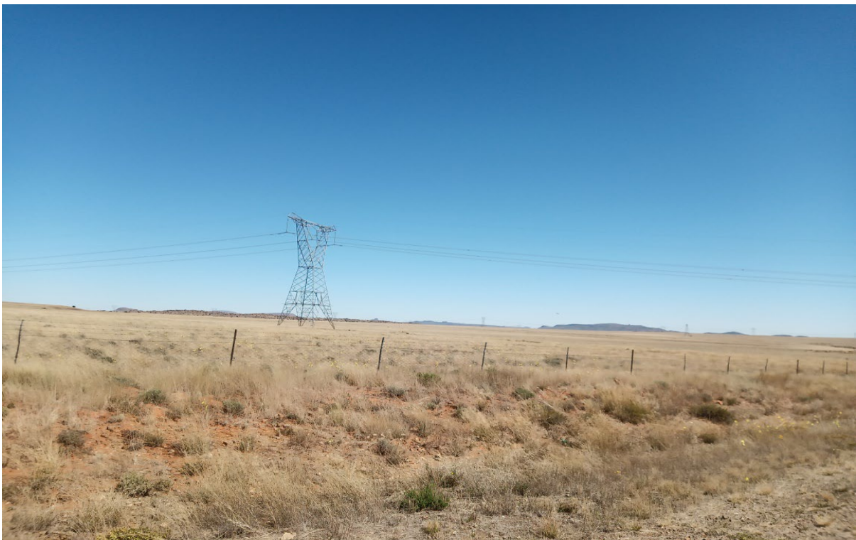
Figure 46: electricity pylons on site
