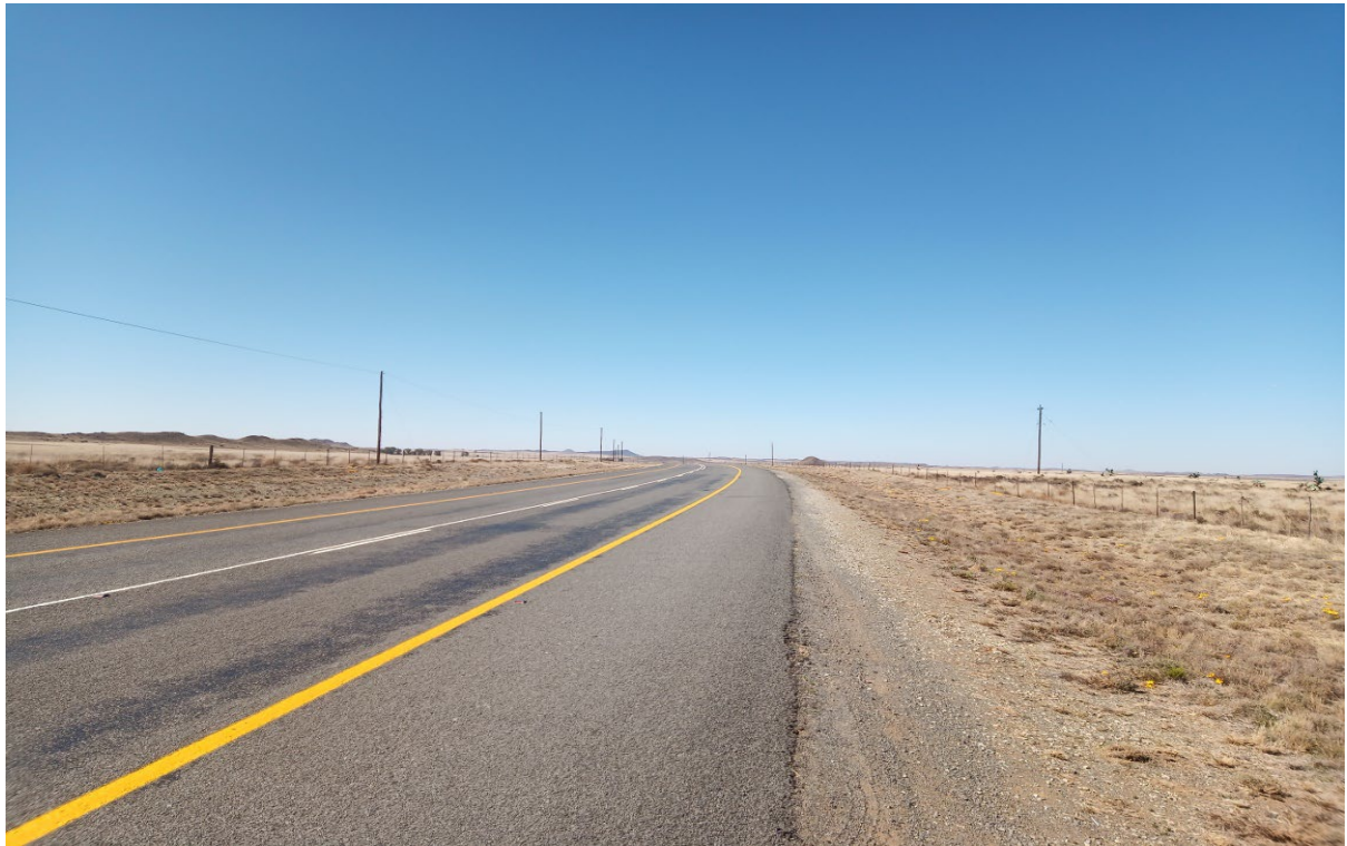
Figure 35: View from the N10 looking southeast
