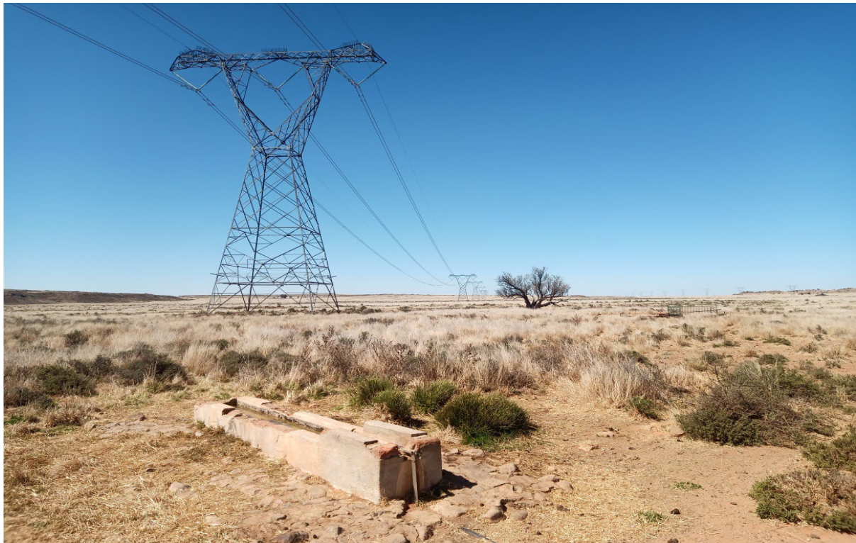
Figure 61: typical site view
