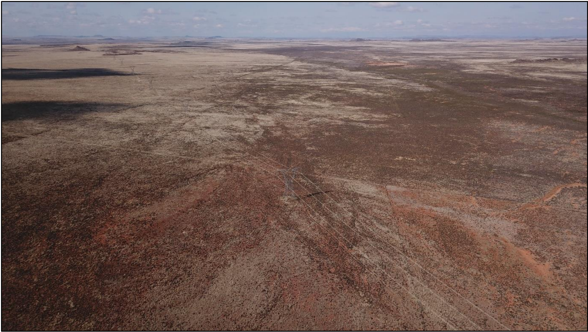
Figure 5: Existing transmission lines.
