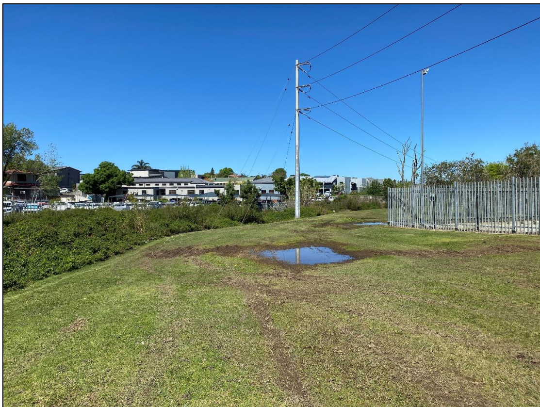
Figure 4-2: Commercial area and fence of an electrical substation (righthand side) flanking the site just upstream of C.J. Langenhoven Road.
