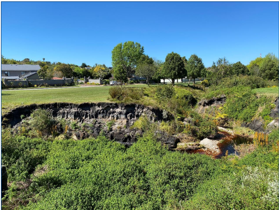
Figure 5-5: Eroded section of the Camfersdrift River inside Van Riebeeck Gardens.
