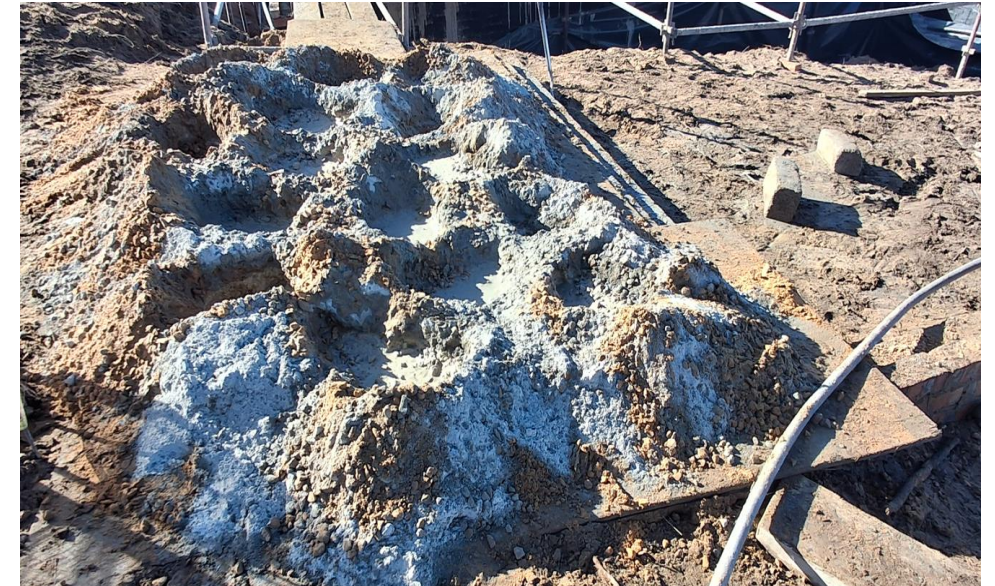
Cement batching on impermeable surface
