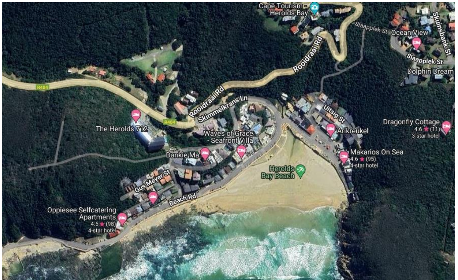
Herold' Bay Pump station and pipeline
