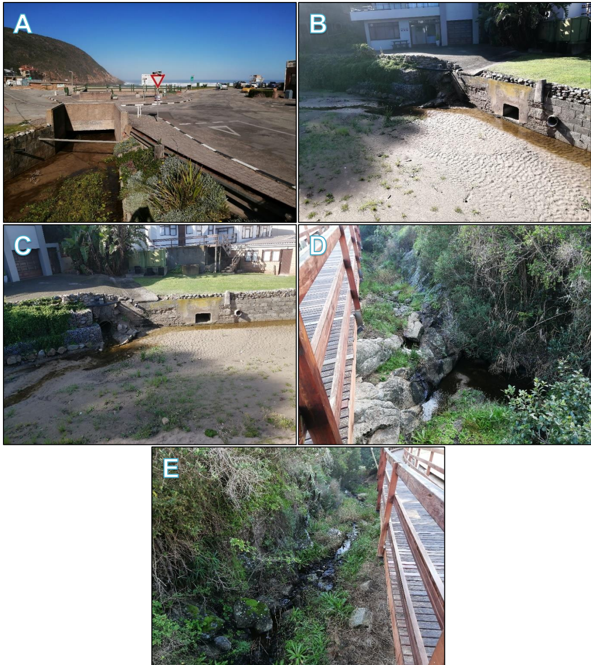
Figure 8: Photographs indicating the existing rising main crossing the estuarine zone (A); marine sediments and bank stabilisation along the edge of the estuarine zone (B and C); bedrock and boulder substrate along the non-perennial watercourse (D and E).
