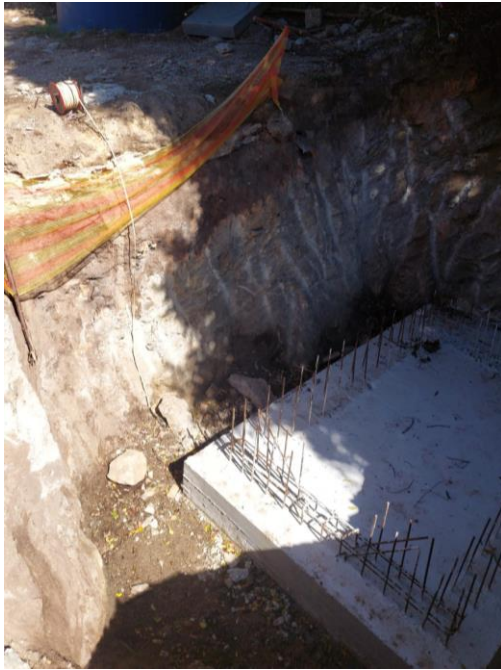
Figure 6. On-site excavation pit showing the absence of shallow groundwater.
