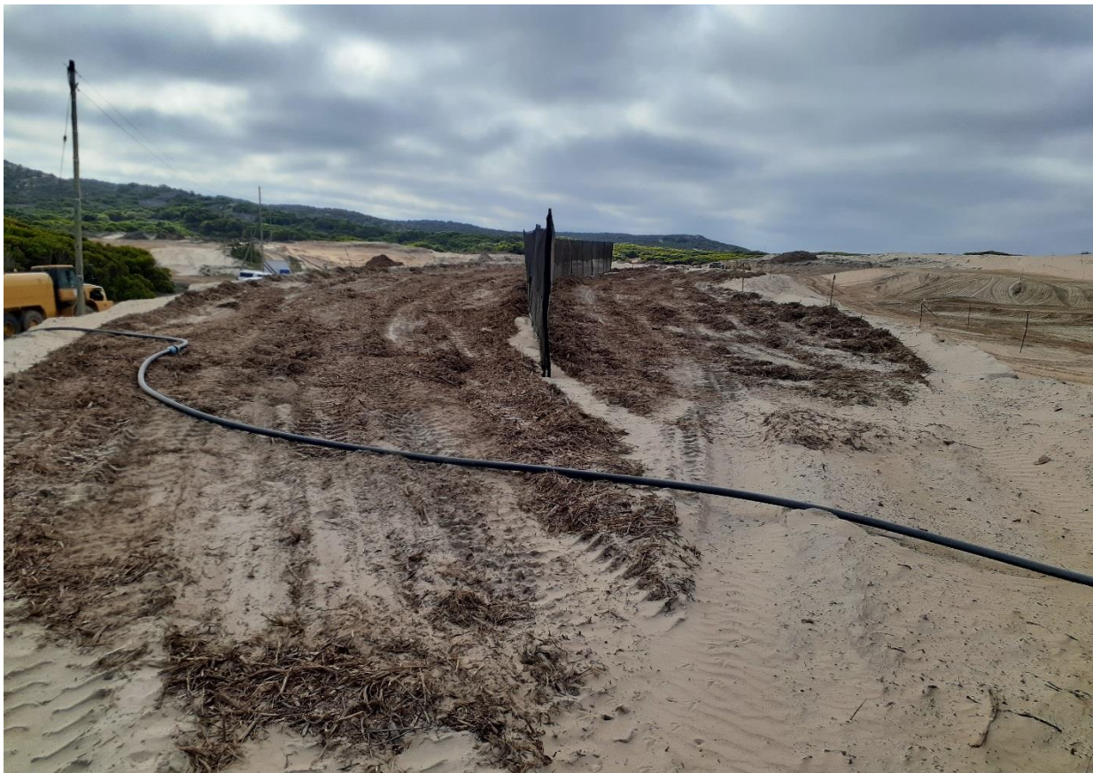
Photo 8: The completed platform for the group housing complex to the south of the entrance to the development. Note the spreading of topsoil and wood chips to prevent windblown sand.
