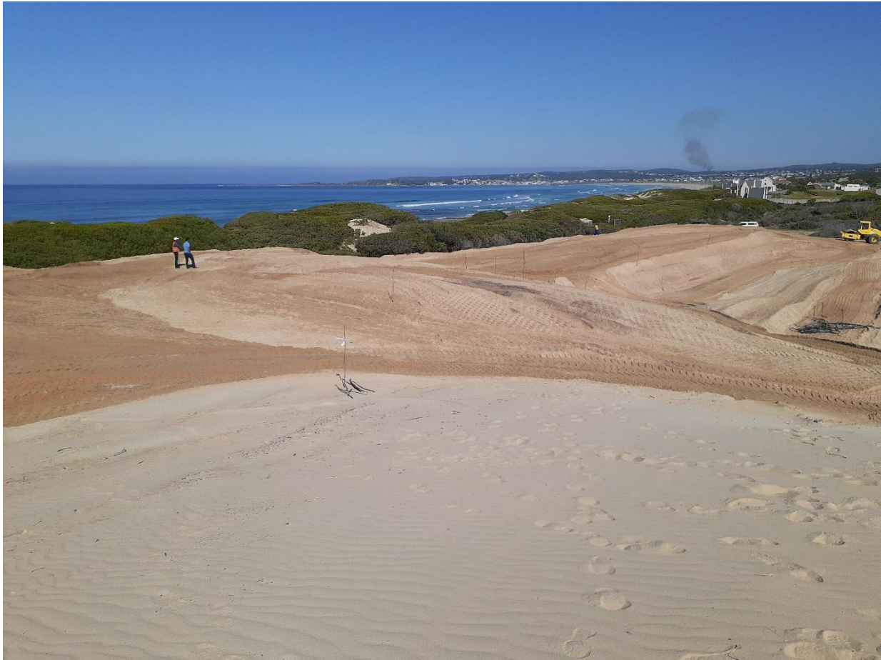
Photo 7: Shows the completed platform for the hotel site (right of photo) and the frontal platform for the first row of houses. The area to the right is private open space which will also include a shallow dam.
