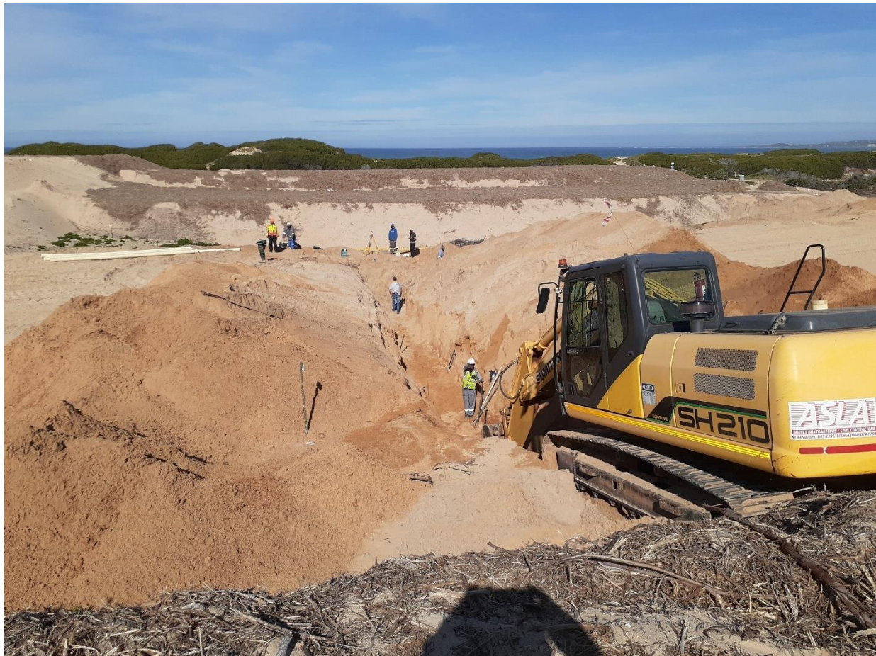
Photo 3: The installation of sewer pipes in the center of an internal road.
