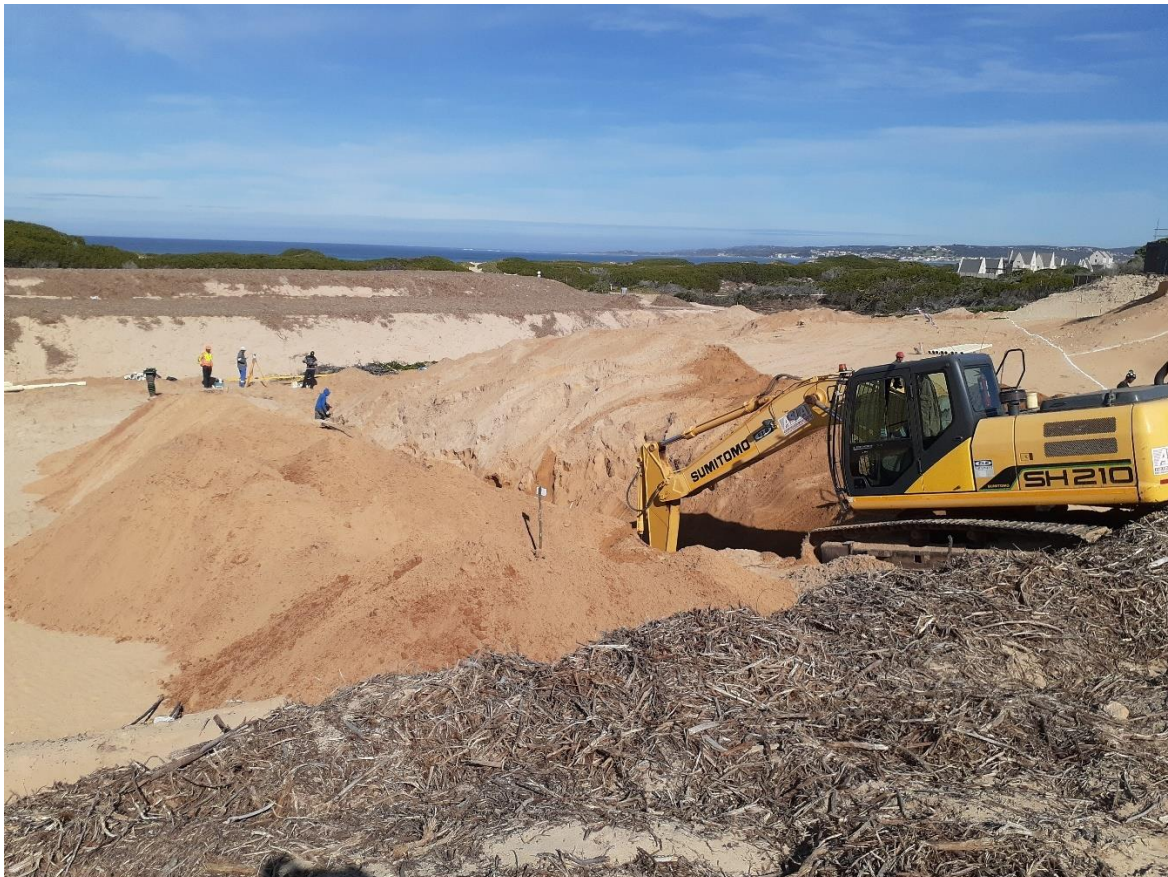
Photo 2: The installation of sewer lines for the Preekstoel Beach Lifestyle Estate. Note the stabilized building platforms covered in wood chips.
