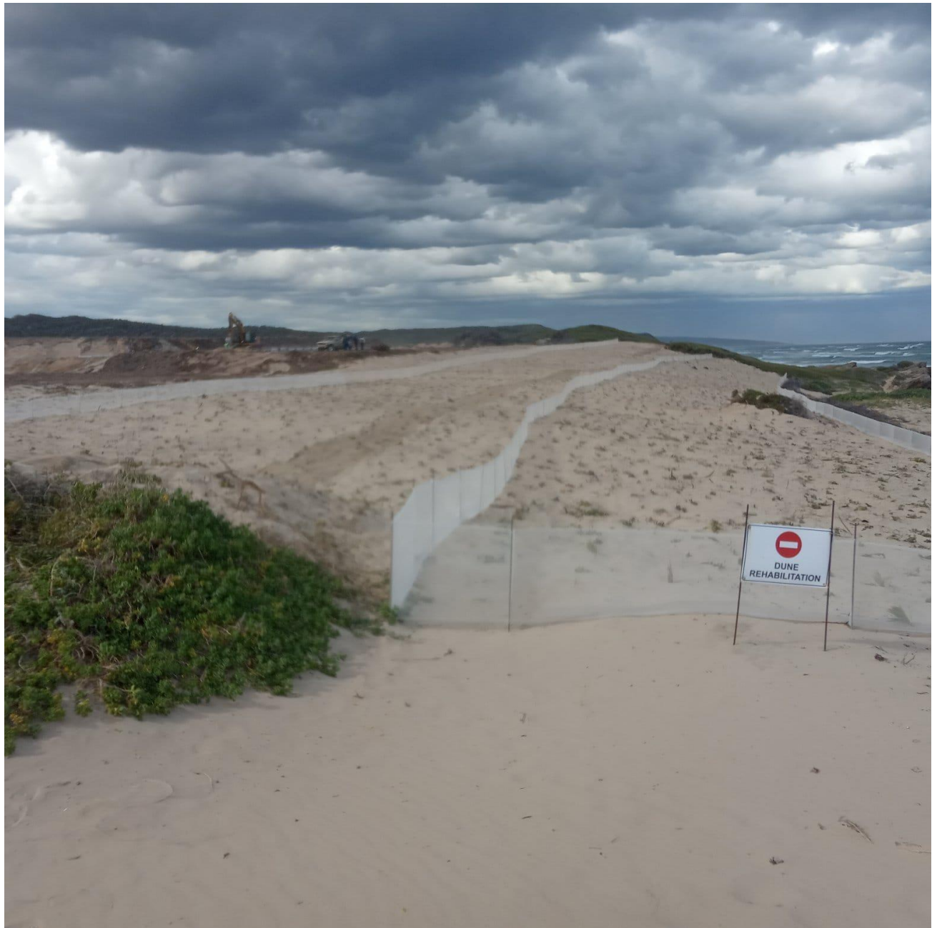
Photo 5: The sand from the unstable back dunes was moved towards the seashore at an angle of repose of dry sand (about 26^\circ ). Note the netting to reduce wind erosion and the soil saver hessian to the left of the middle net. The whole area was planted with indigenous strand plants about 1m apart.
