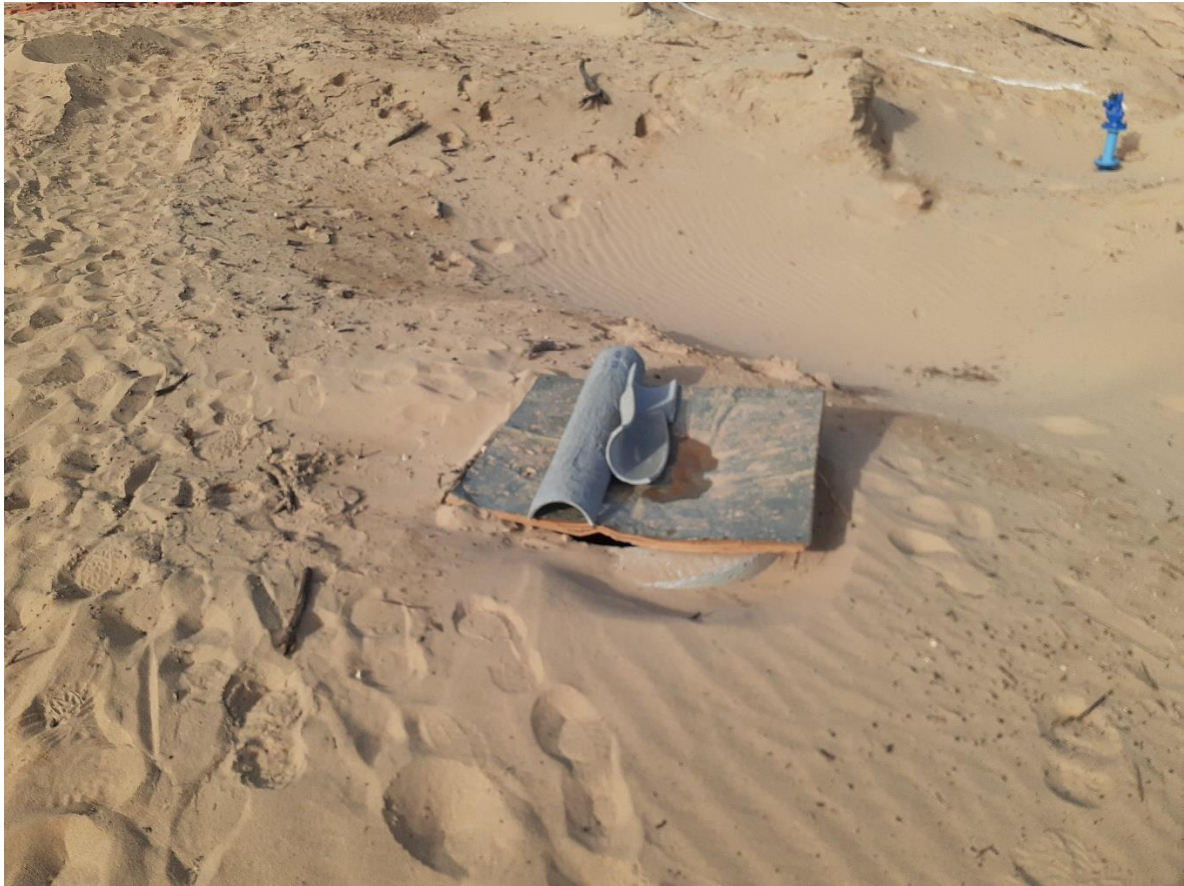
Photo 7: The manhole must have stakes around it and danger tape around the stakes.
