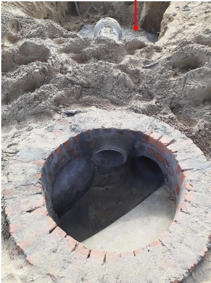
Photo 3: The use of concrete (red arrow) and brickwork on site for stormwater drainage.
