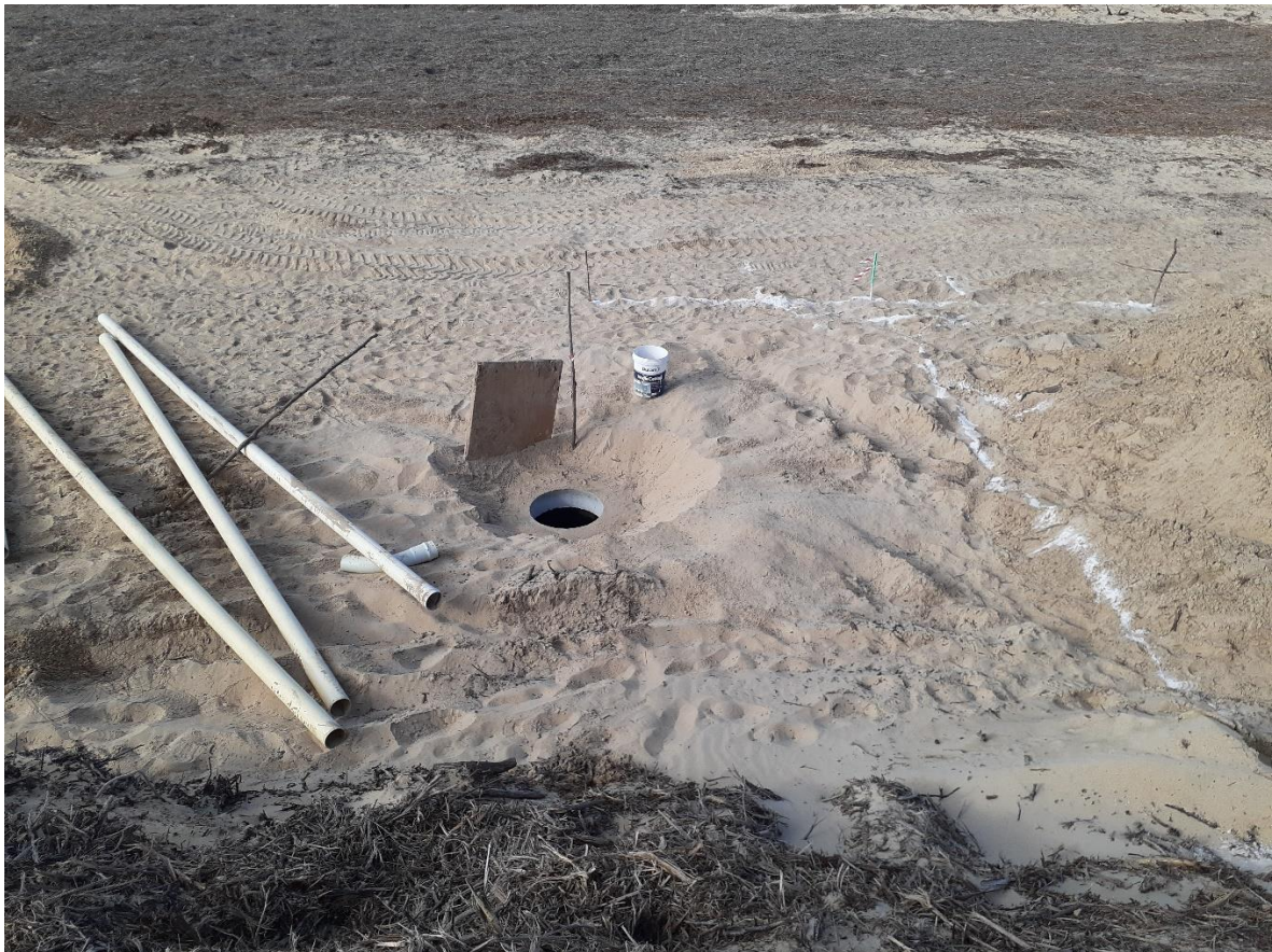
Photo 8: Open manholes must be demarcated with stakes and danger tape. Sand should also be prevented from entering sewage manhole.
