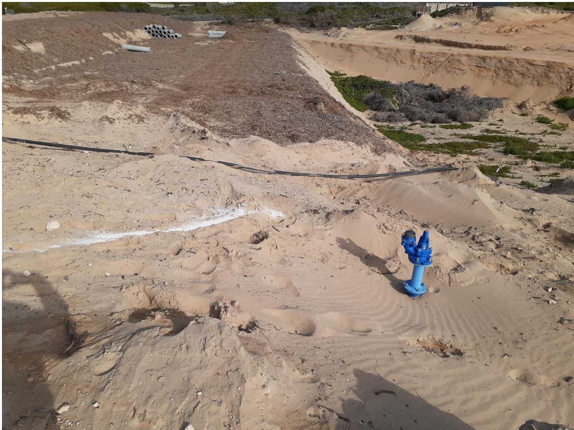
Photo 4: Potable water pipelines and pressure release valves are being installed. Note the small stormwater detention pond in top right corner of photo.
