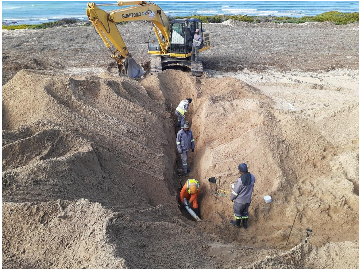
Photo 5: The laying of sewage pipes to individual erven.
