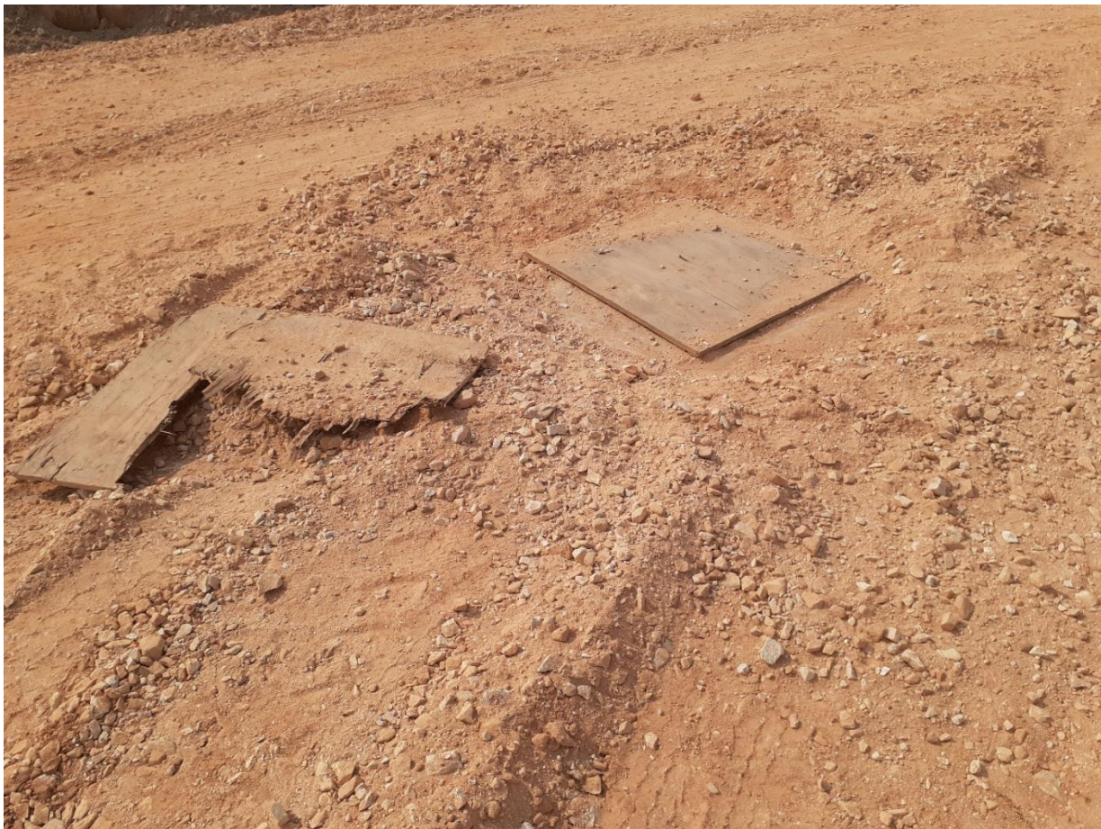
Photo 10: The manhole must have stakes around it and danger tape around the stakes.
