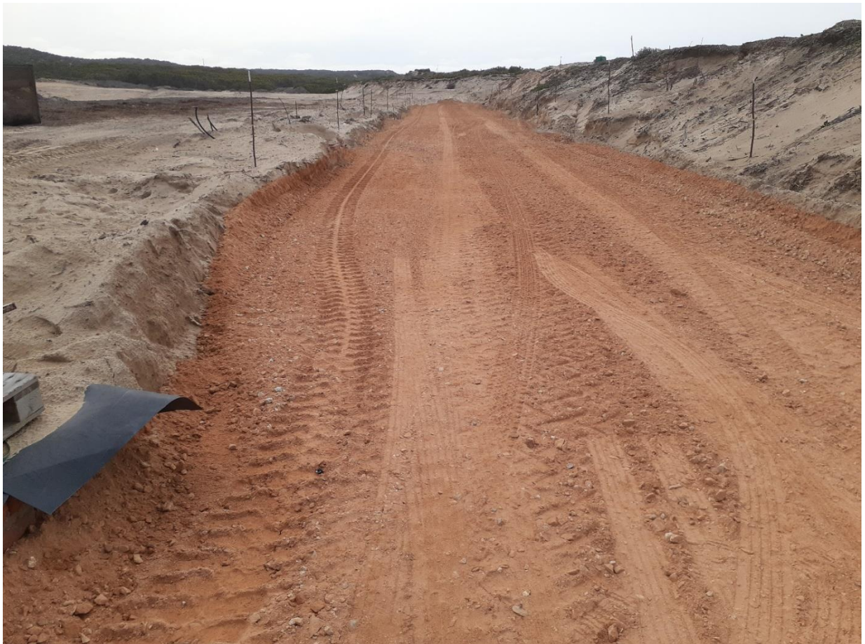
Photo 8: Internal roads are being constructed for Phase 1 of the development. G5 material is being spread and compacted.
