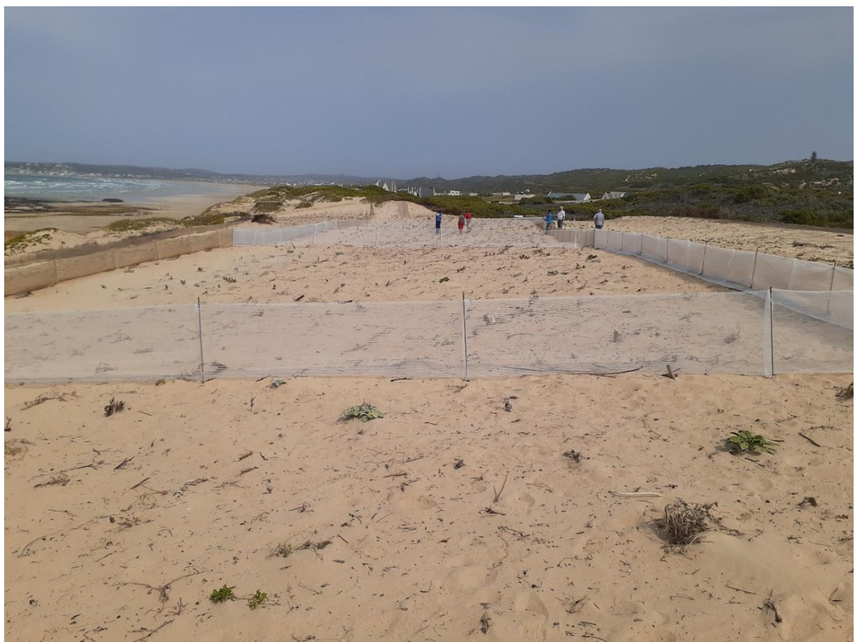
Photo 6: New internal netting has been erected within the rehabilitation area to prevent windblown sand. Note the growth of locally planted strand plants.
