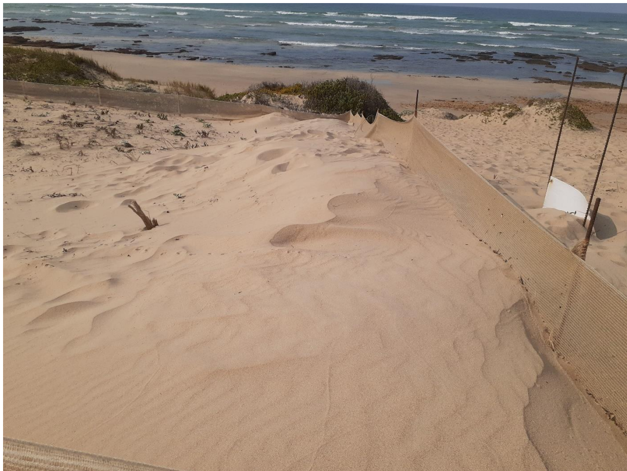
Photo 5: Windblown sand has accumulated to the west end of the dune rehabilitation area.
