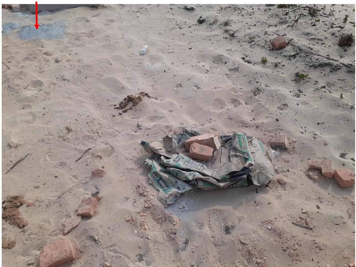
Photo 4: Cement packets must be placed in dustbins. Cement powder spills must be picked up (arrow). Plastic wrapping is also to be picked up.
