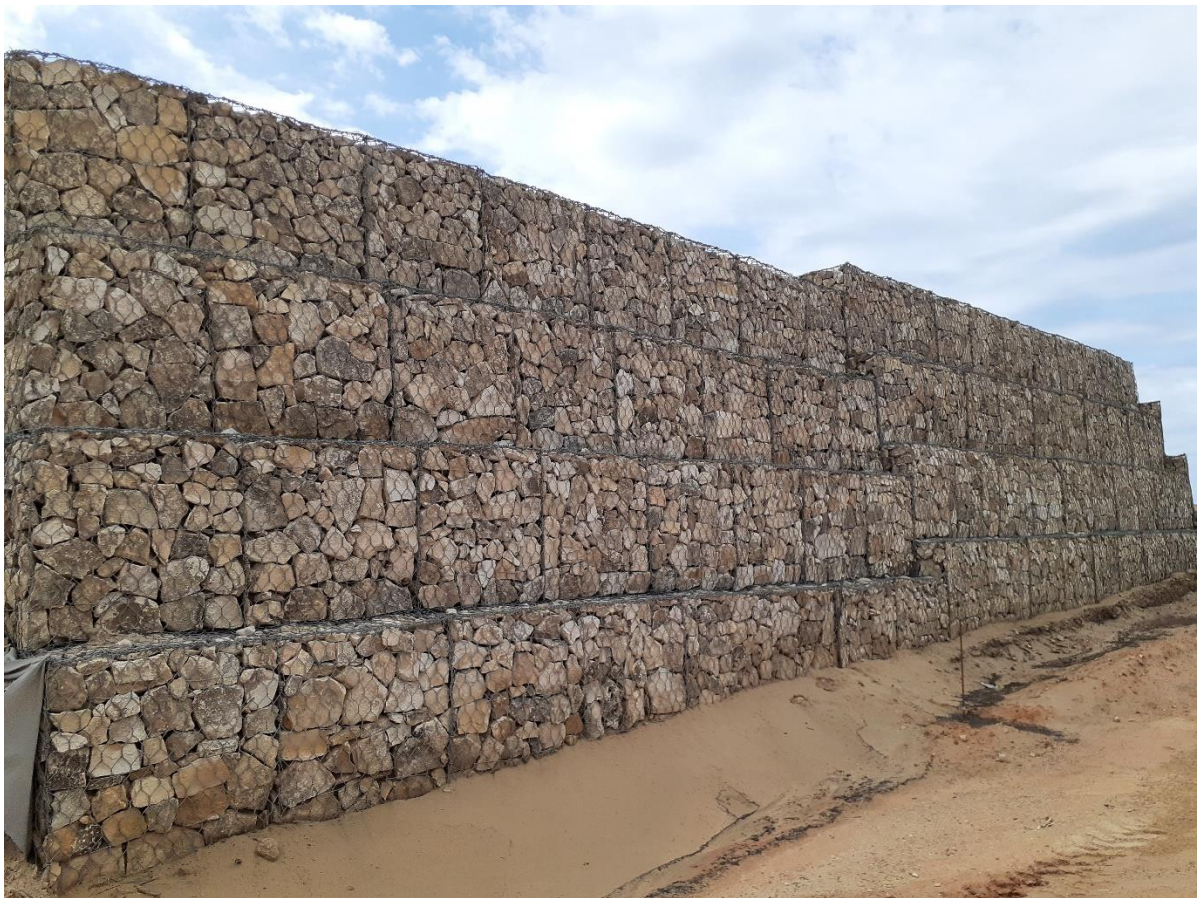
Photo 4: The gabion retaining walls have been completed for the first phase of the project.
