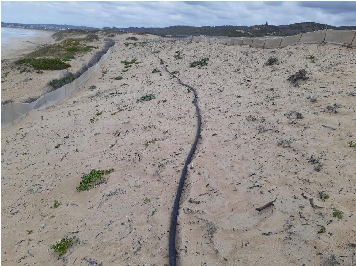
Photo 3: A temporary irrigation system has been installed on the rehabilitated dune system.
