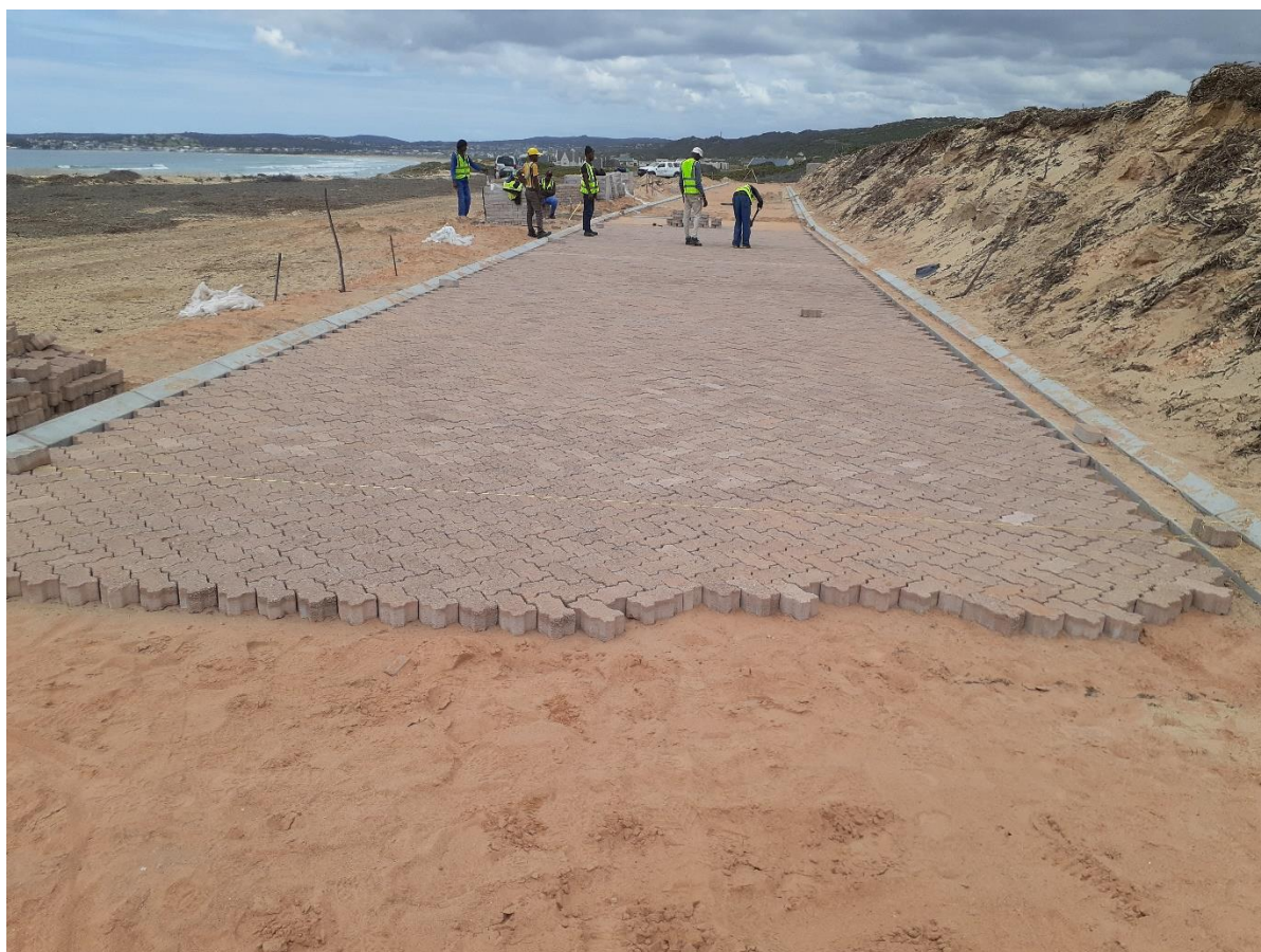
Photo 6: Paving of the internal roads are also being undertaken.
