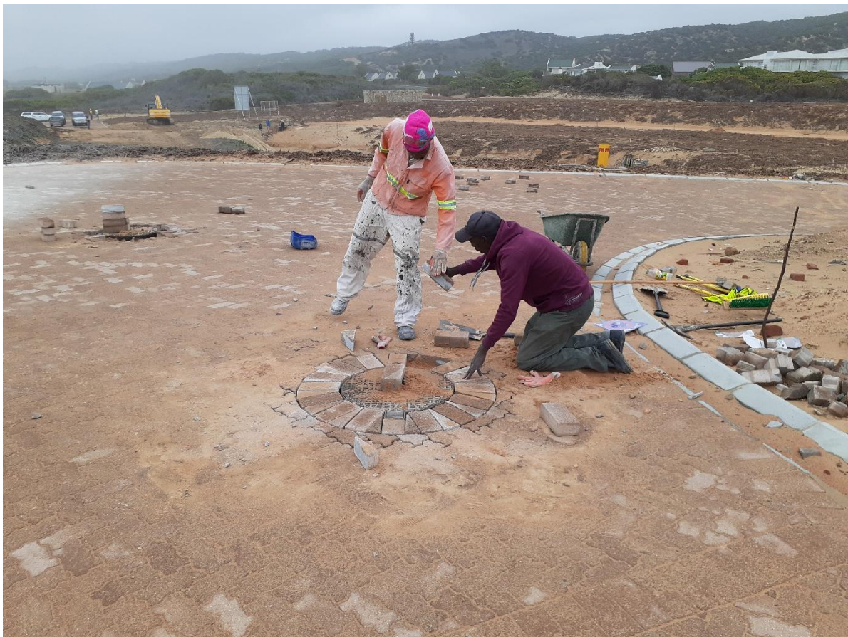
Photo 8: The manholes were all in place and the final paving was being undertaken around such manholes.
