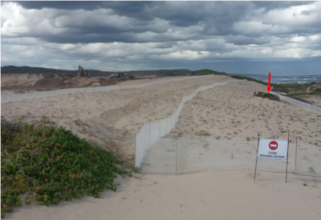
Photo 2: Photo 1 was taken at approximately the same place as Photo 2. Photo 2 shows the rehabilitated frontal dune as on 21 August 2022. The red arrow shows the top of the same “stack” as in Photo 1. The stack was about 3.5m high. The transplanted strand plants can be seen between the shade cloth “fences”.
