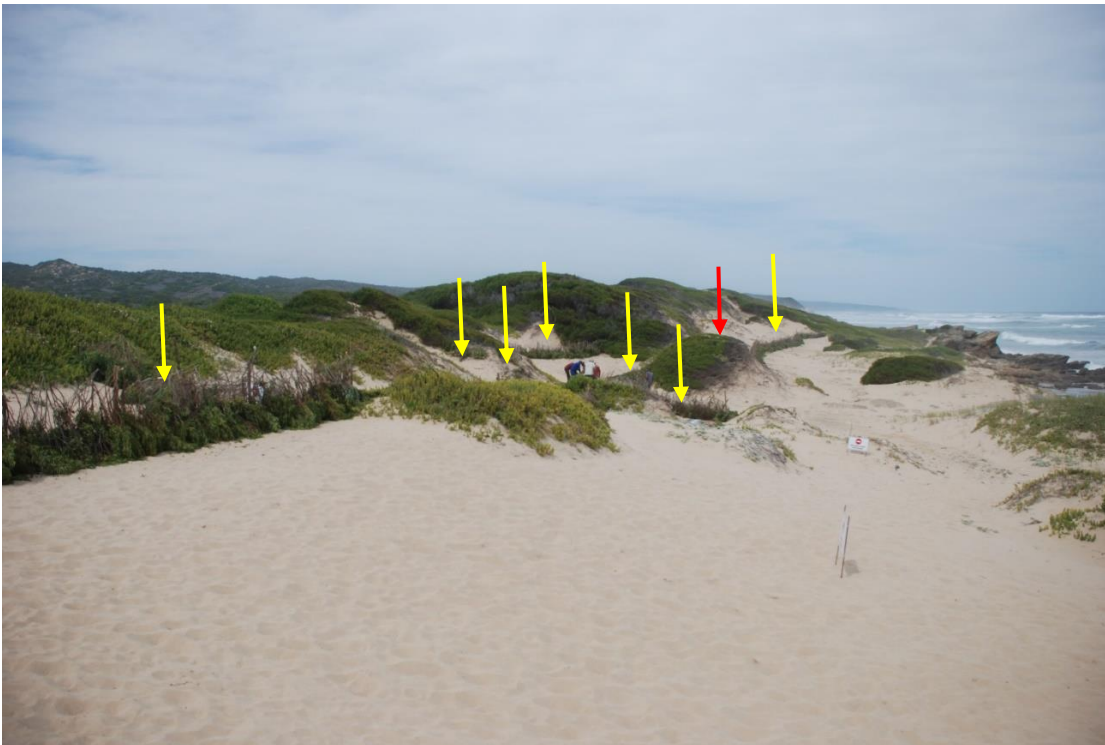
Photo 1: About 220m of brushwood fencing (arrows) was erected on the highly eroded Preekstoel frontal dune system.
