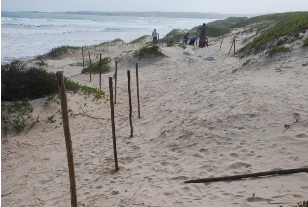
Photo 4: The layout of poles where sever wind erosion has taken place. Three strands of wire is attached to the poles about 1m off the sand.
