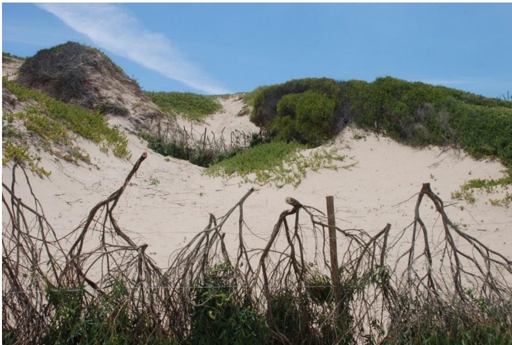
Photo 7: The brushwood was weaved between the wire strands and fixed to the wire with binding wire. Not the large blow-out towards the back of the dune. A brushwood fence has been placed in the blow-out to trap windblown sand.
