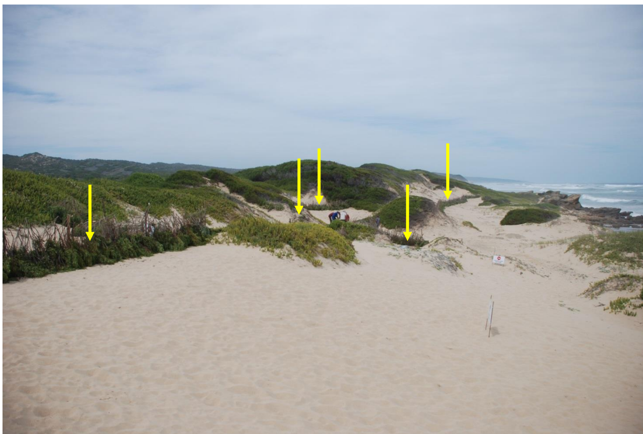
Photo 8: About 220m of brushwood fencing (arrows) has been erected on the highly eroded Preekstoel frontal dune system.
