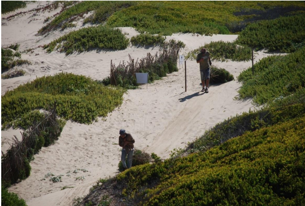
Photo 6: Brushwood was dragged to the areas where brushwood fences were erected. Note the brushwood fences to the left of photo.
