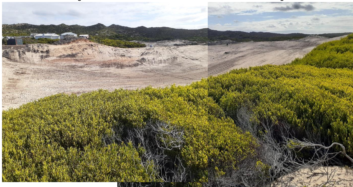
Photo 8: The entire site has been de-grubbed
