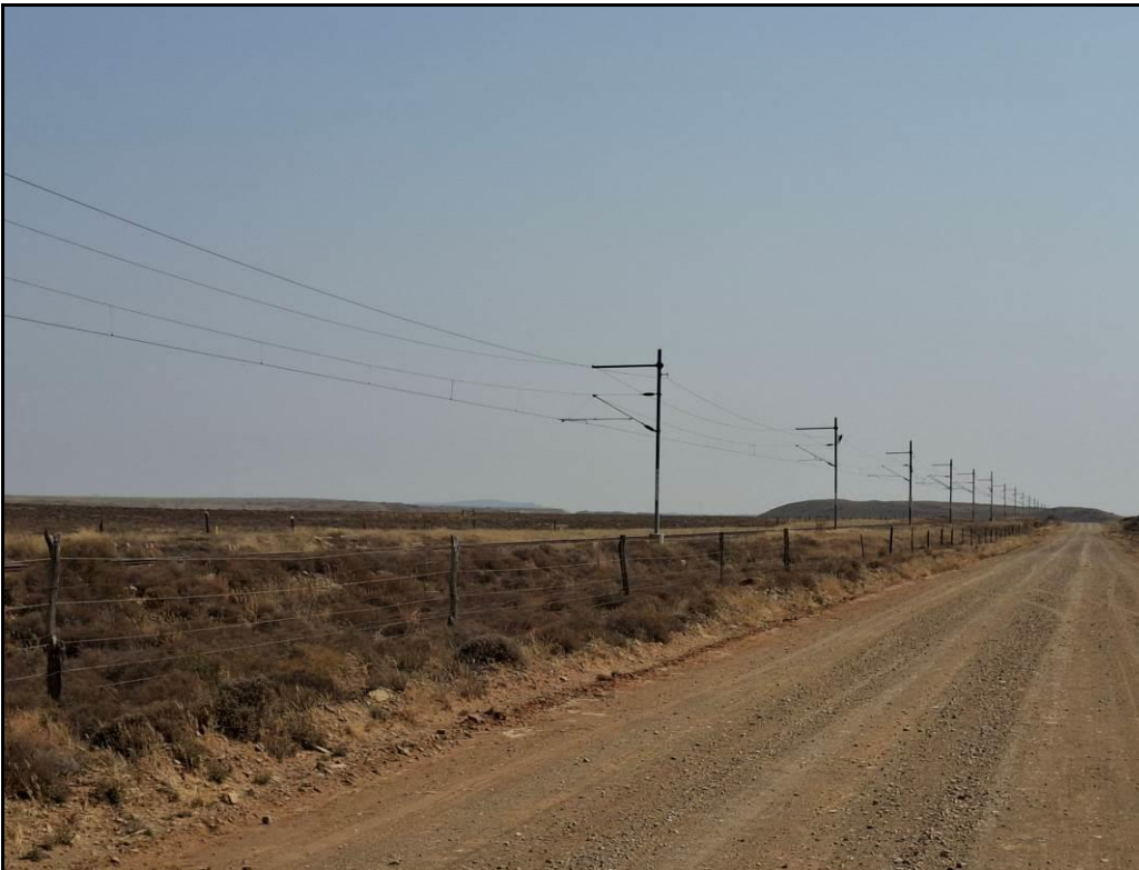
Photograph 3.2: Railway line and service road to the north of the study area
