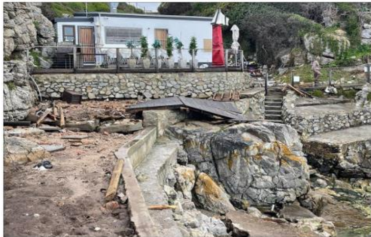
Figure 3 depicting the damage of the September 2023 storm event with the wooden decks, furniture and balustrade completely destroyed
