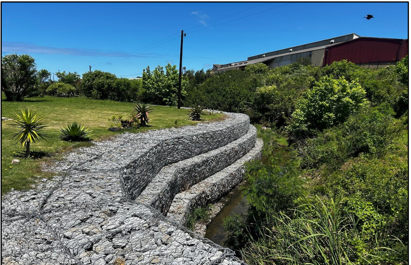
Image 1: Gabions that have been installed.
