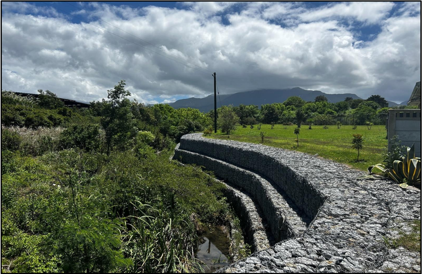
Image 2: Gabions that have been installed.
