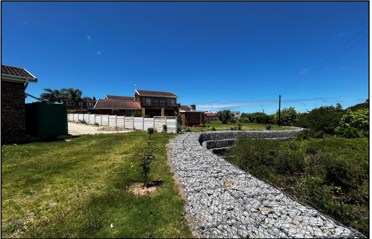
Image 8: Gabions that have been installed and work area that has been rehabilitated.
