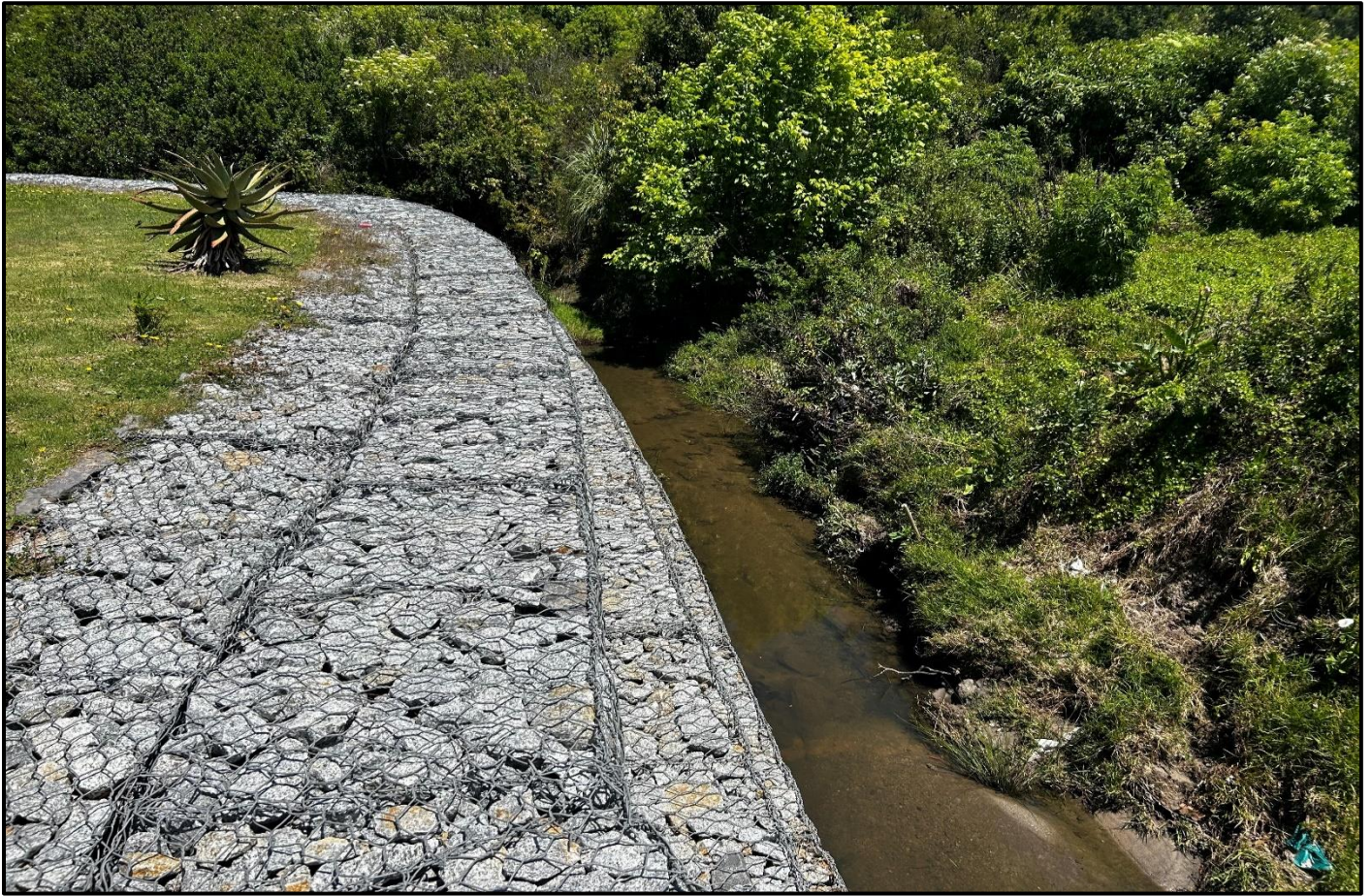
Image 6: Gabions that have been installed and kweek grass that has been planted.
