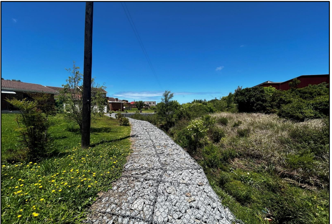
Image 9: Gabions that have been installed and work area that has been rehabilitated.
