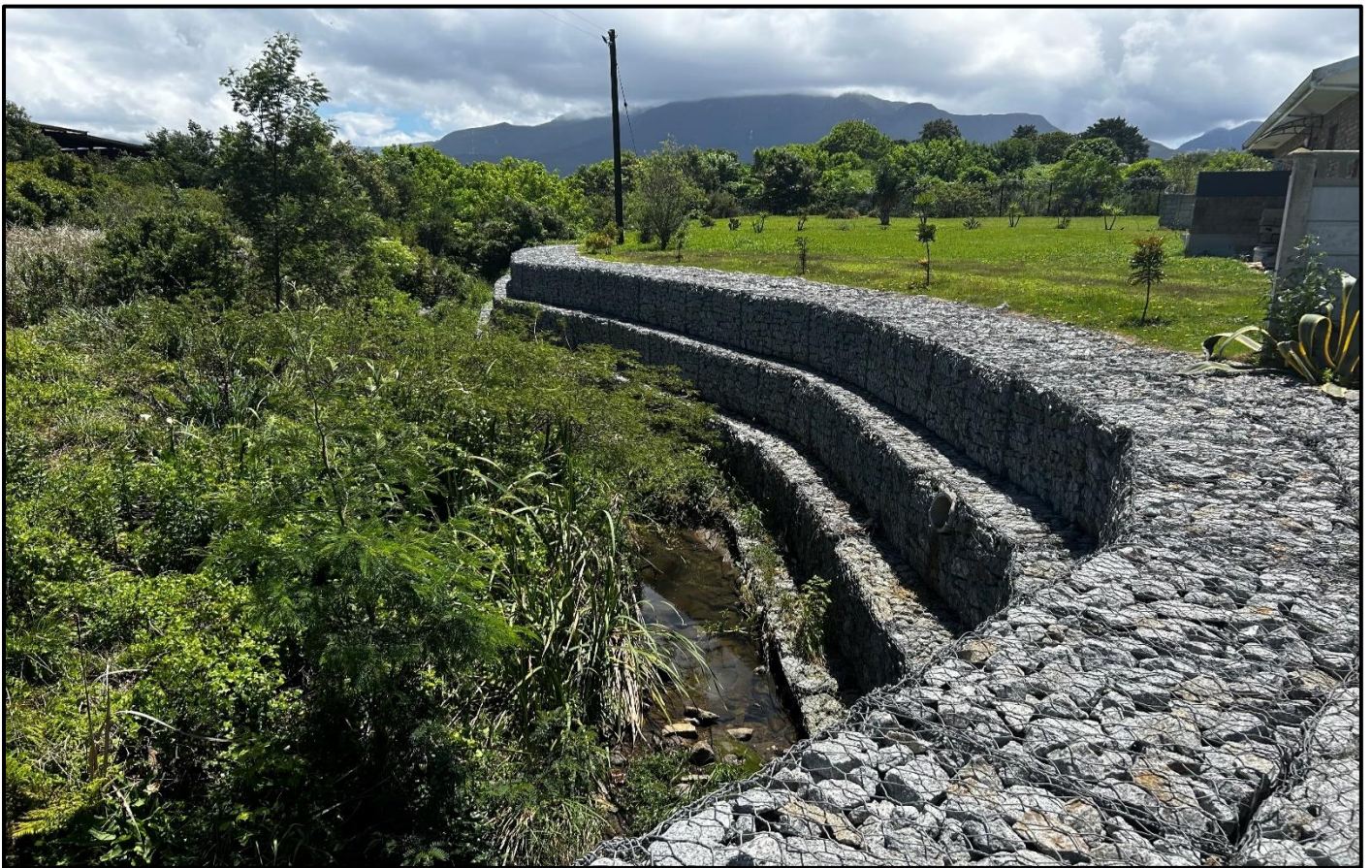
Image 5: Gabions that have been installed.
