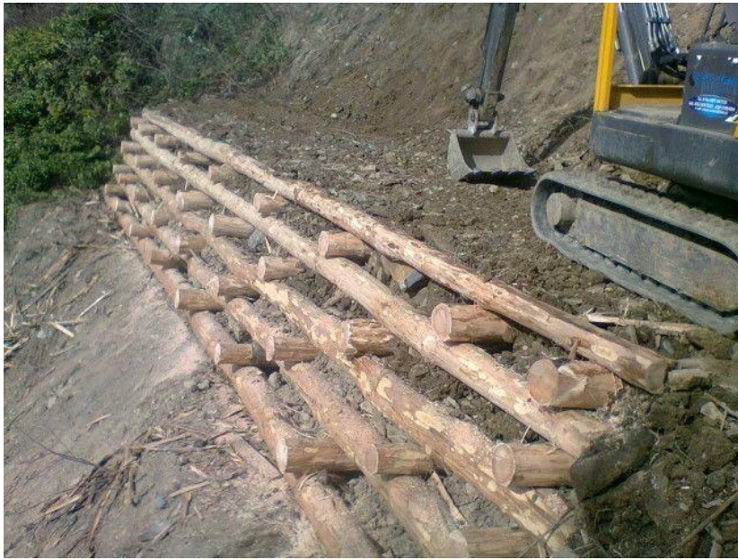
Figure 15 – Timber log terrace fill for slope control and protection.
