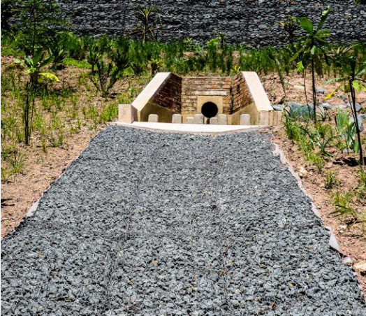
Figure 26 – Accepted general outflow structure erosion protection systems that are implemented in practice against slopes.
