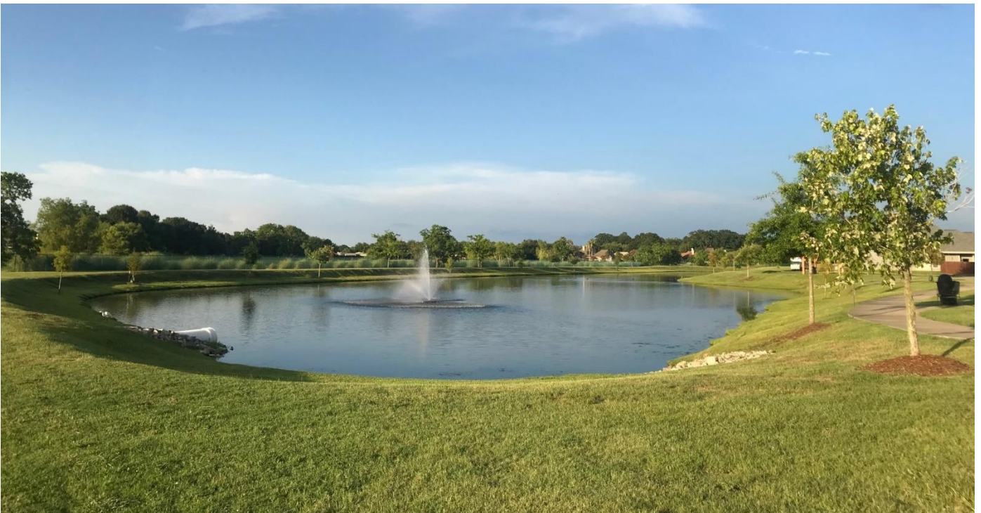
Figure 9: Typical depiction of an attenuation pond with floating fountain.
