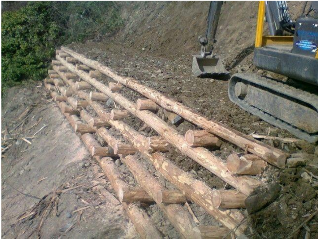
Figure 8: Timber log terrace fill for slope control and protection.
