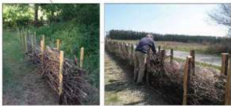
PROPOSED PACKED BRUSH FENCE 2m FROM RIVER BANK TO PROTECT REHABILITATION PLANTING
