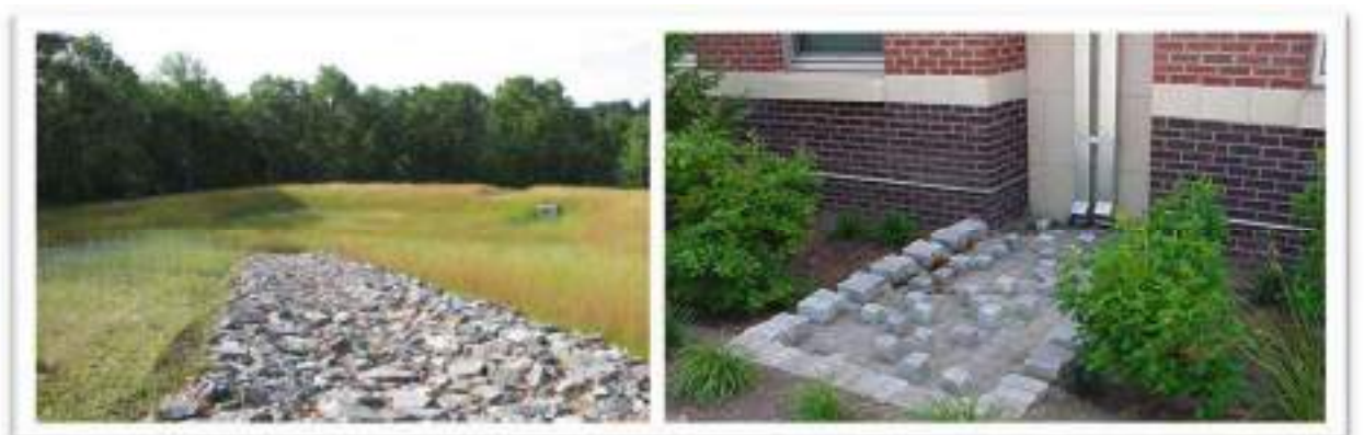
Figure 2-4 Energy Dissipaters
