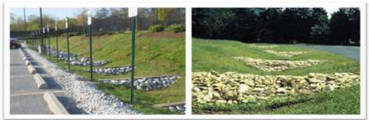
Figure 2-3 Examples of Stepped Energy Dissipaters
