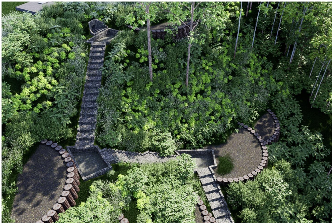
Figure 20: Outflow Headwall structure into 1st stilling pond, followed by 1st water stair section to the
