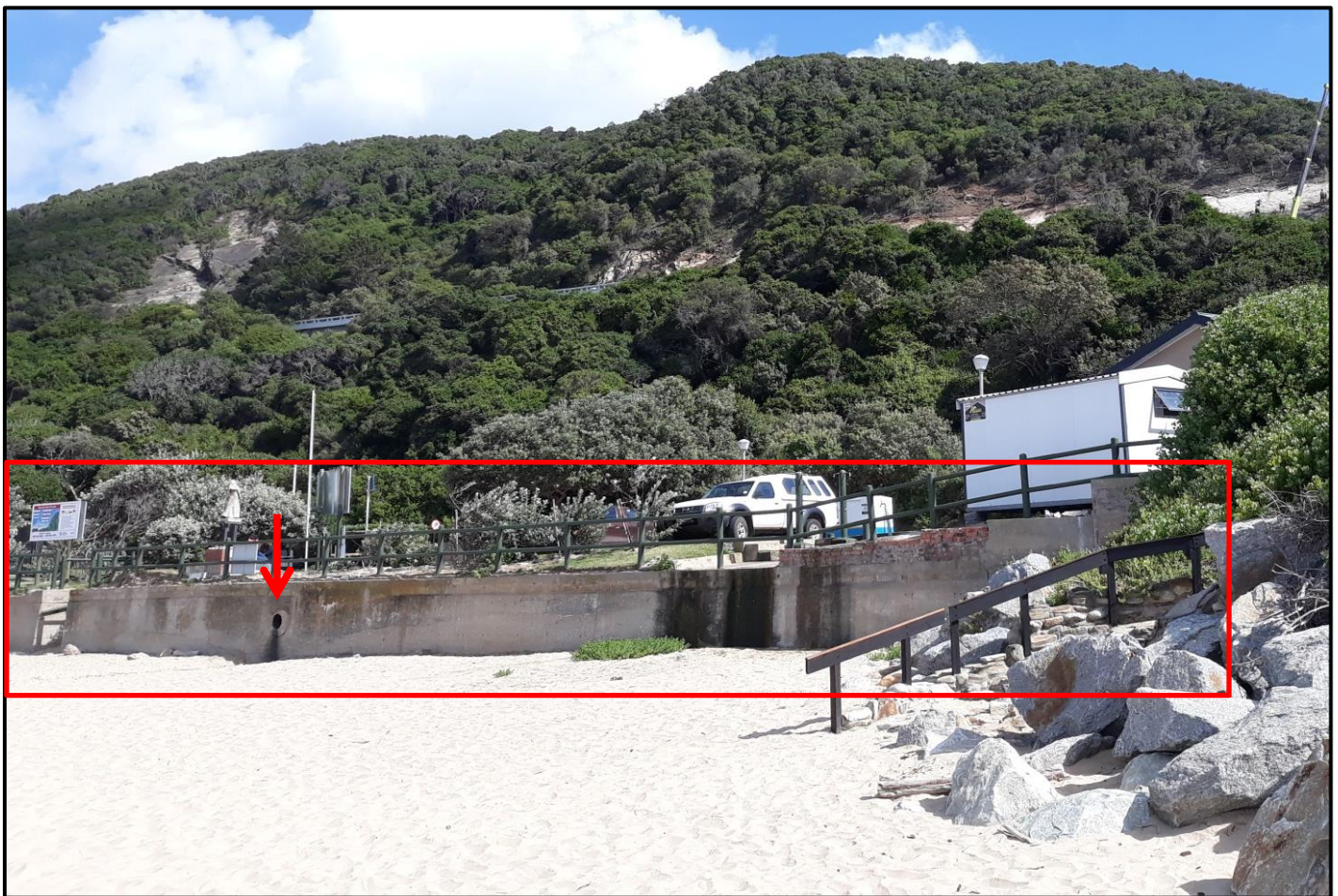
Figure 9 The concrete revetment wall of the Wilderness Beach Front. Note the small pipe (arrowed) which is used to channel the drainage of the western non-perennial drainage channel onto the beach.
