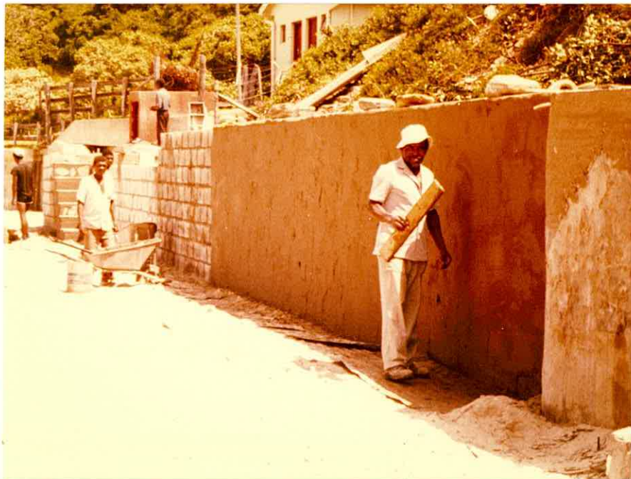
Photo 16. Final plastering of the wall.
