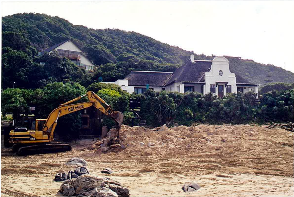
Photo 47. This shows the Front End Loader placing the final few rocks in place and covering them with a layer of beach sand.
