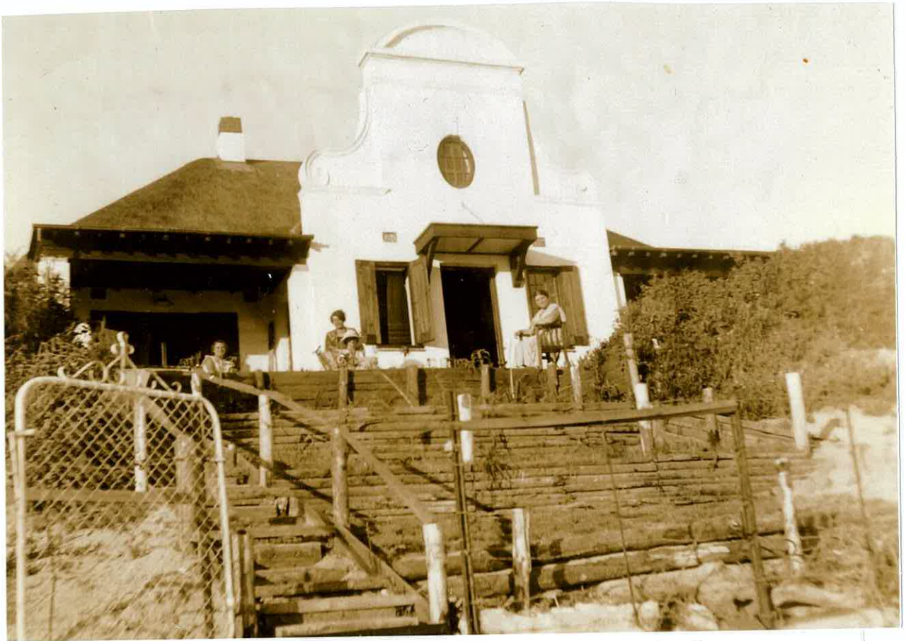
Photo 5. Circa 1934: The completed house showing the front terraced sand dune. This was the very first fortification built by my grandfather to protect the house from the sea.
