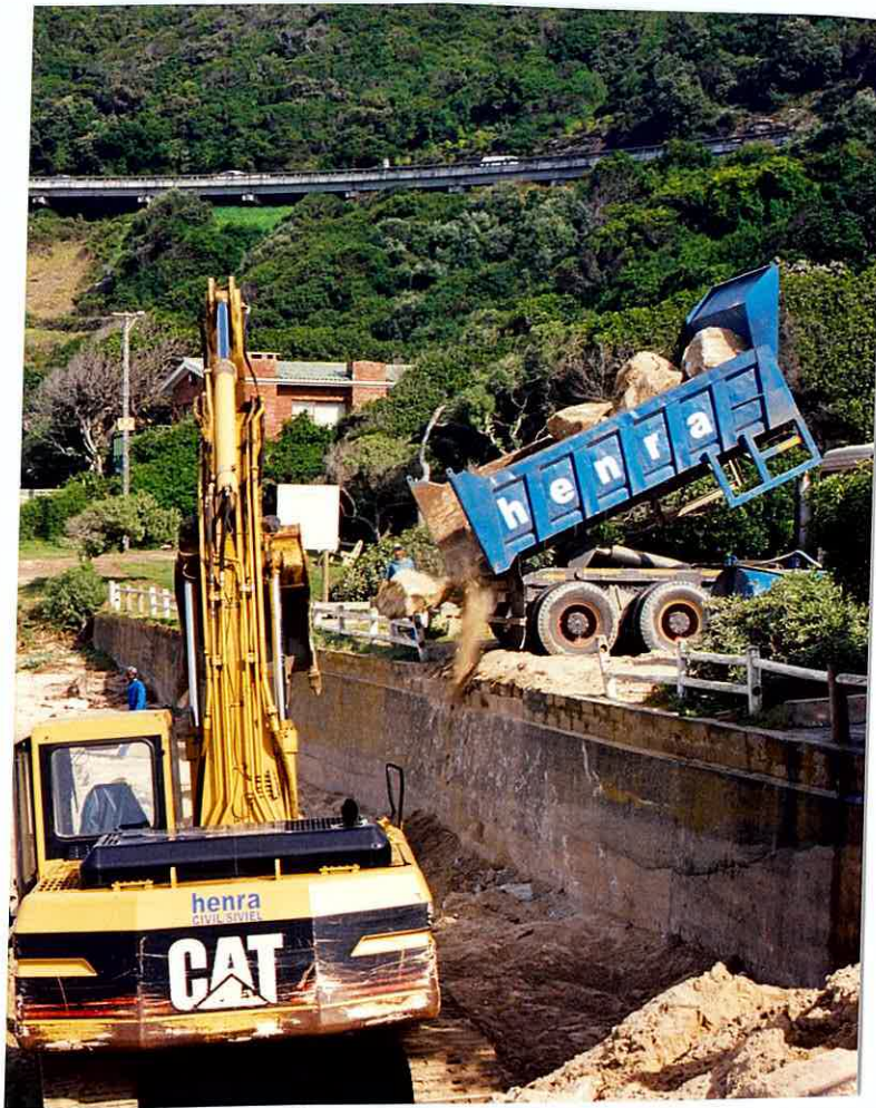
Photo 45. This shows rock boulders being tipped off onto the beach from the Public Car Park
