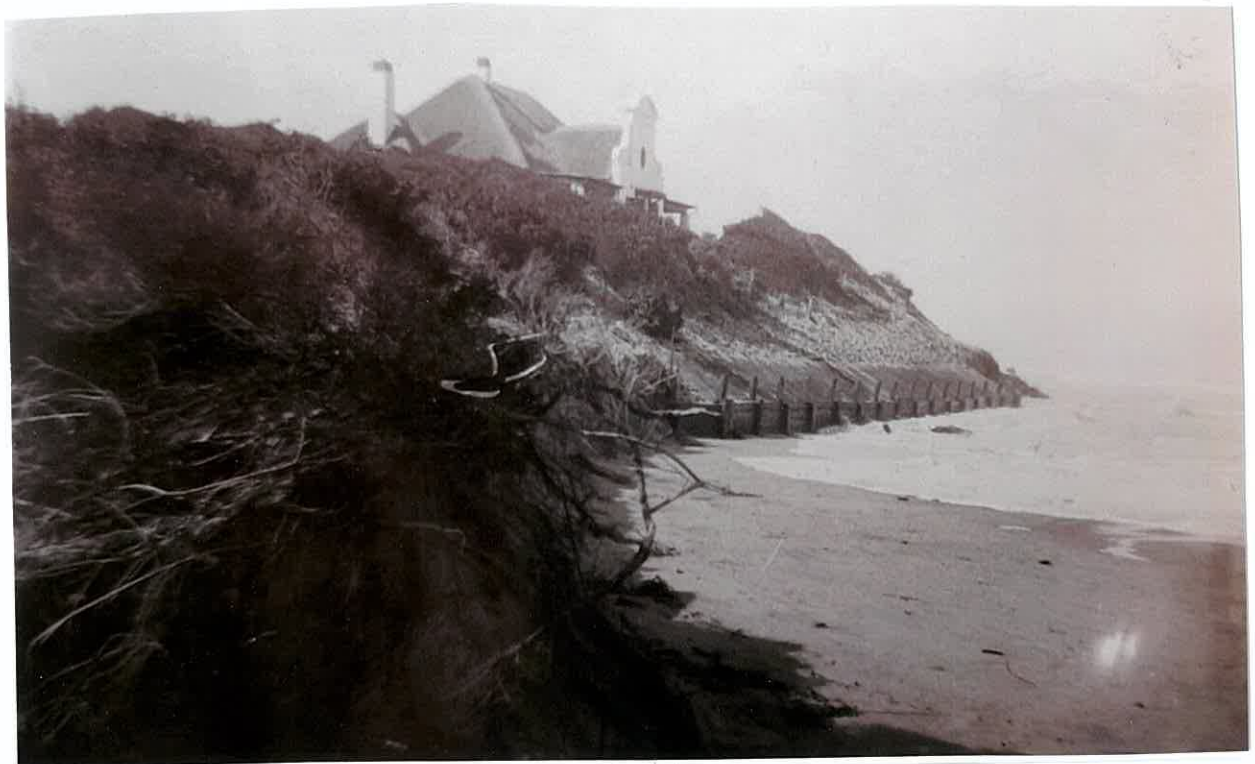
Photo 6. Circa Late 1930's: This side view from the West shows the first substantial barrier of wood being built to protect the house from the sea.
