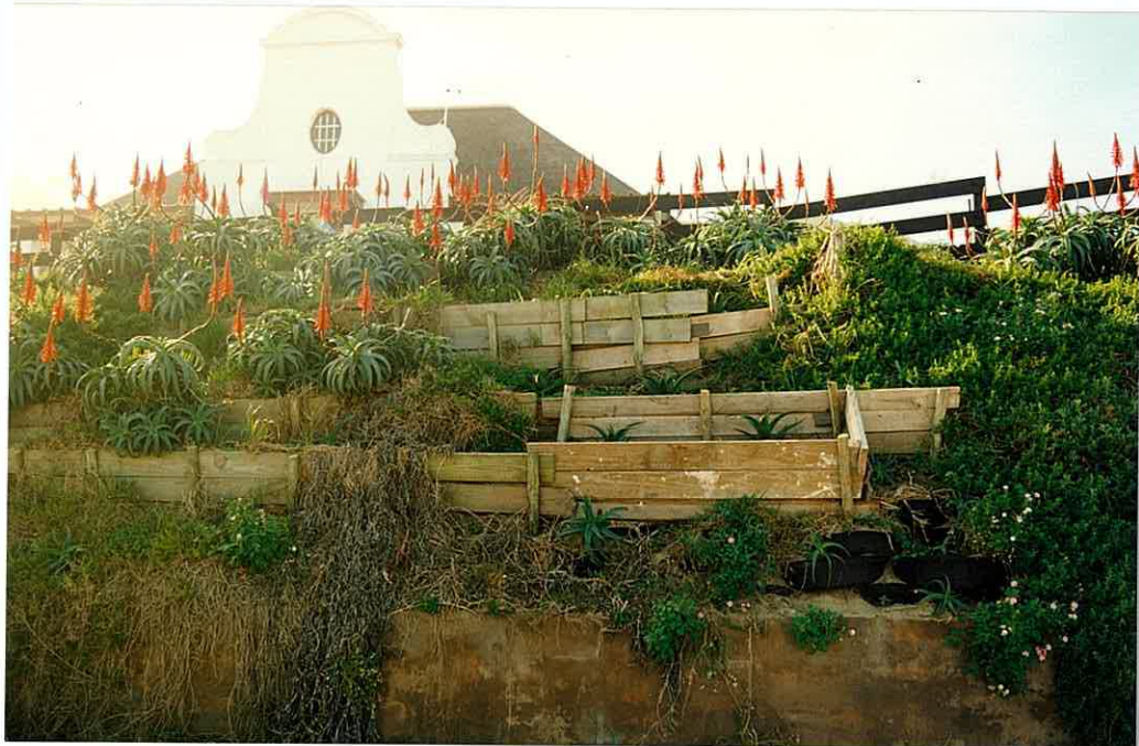
Photo 17. In 1987 the protected terrace behind the wall was backfilled with soil up to the level of the wall. The slope was then terraced and more indigenous plants were added.
