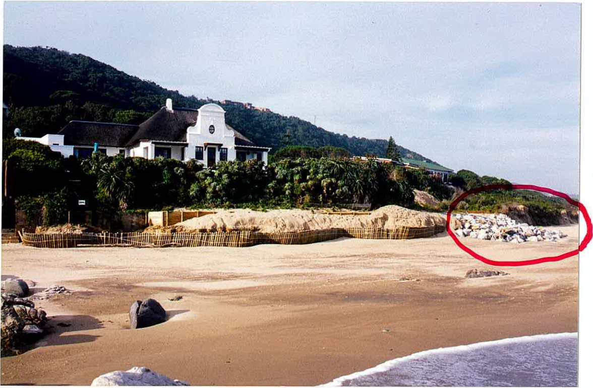
Photo 35. A view from the beach. Here one can see to the right of our pole barrier (ringed in red) is a barrier of rock boulders protecting Erf 91 next to ours.
