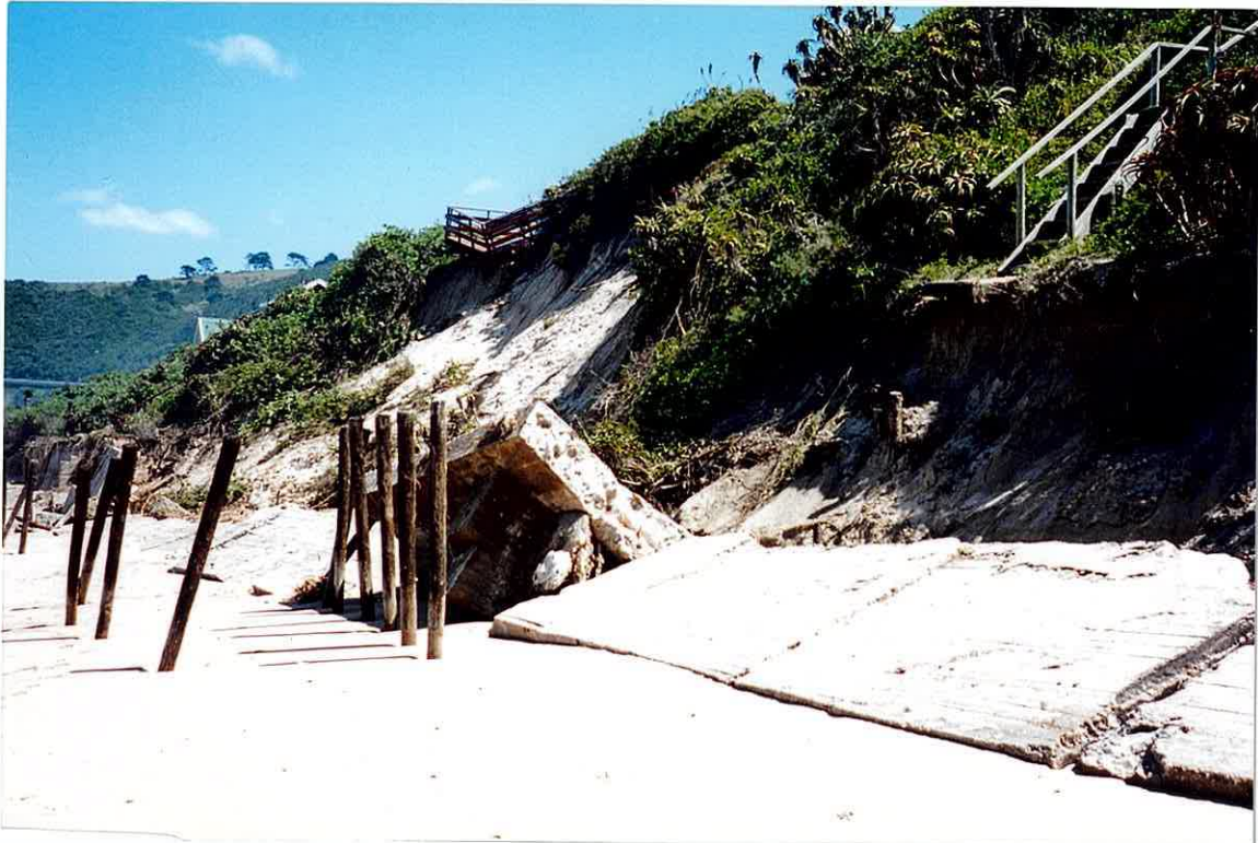
Photo 43. Here one can clearly see the fallen protective wall.
