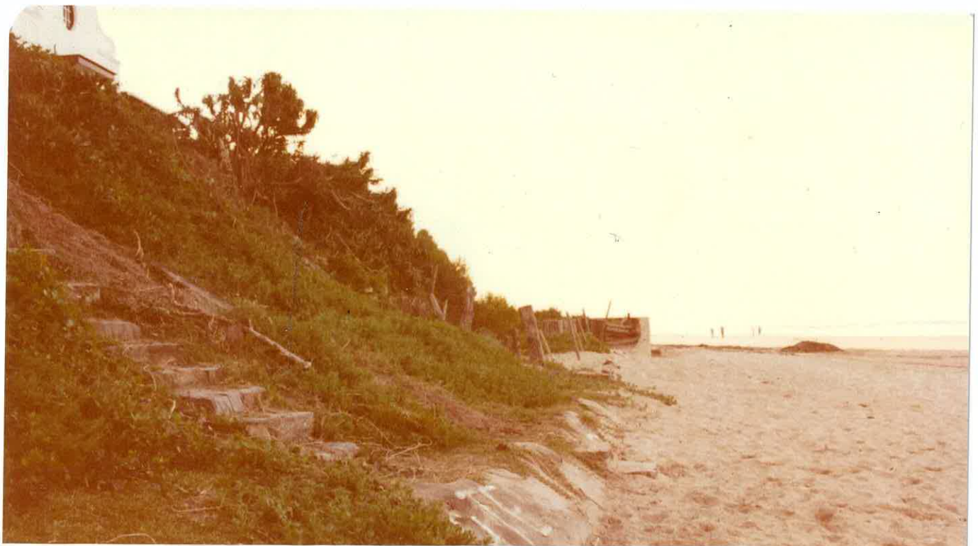
Photo 11: Here we see the first brick and mortar barriers which were built on the property's boundary at beach level to protect the house from the ravishes of the sea. In the foreground is the low sloping dyke built by my grandfather in the early 1960's. Further along is the curved reinforced wall built to protect the more vulnerable South-East portion of the property.
