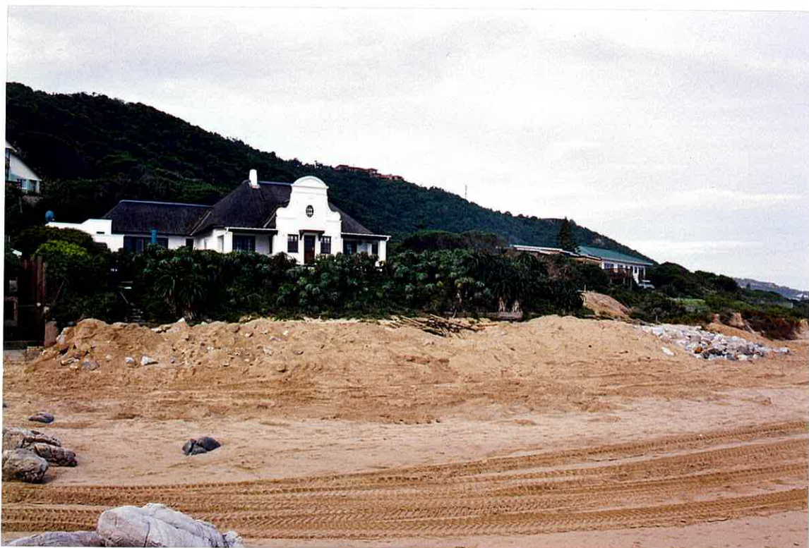
Photo 48. Here one can see the completed rock barrier under a layer of beach sand. The open uncovered rocks on the right of the photo are those previously placed by my neighbour on his Erf 91.
