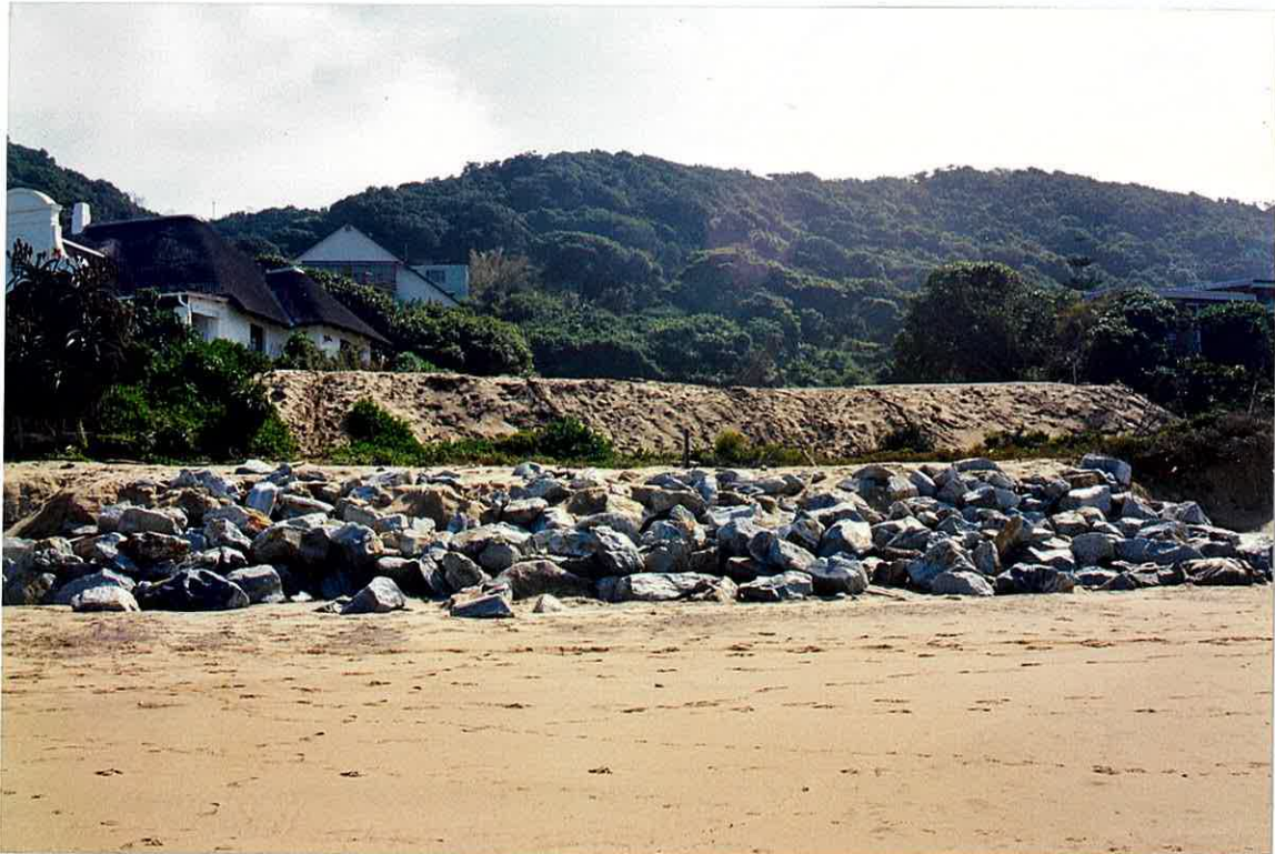
Photo 36. Here one can clearly see the barrier of rock boulders protecting the levelled sand dune of Erf 91 above. Here the Erf had already been prepared for the owner's house to be built. This rock barrier had been installed some years before. I am not sure of when this was done.
