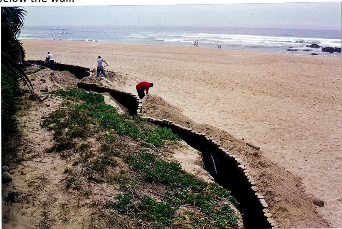
Photo 25. This shows the poles being planted 1,5 metres deep on the boundary between the plant life below the wall and the bare beach.
