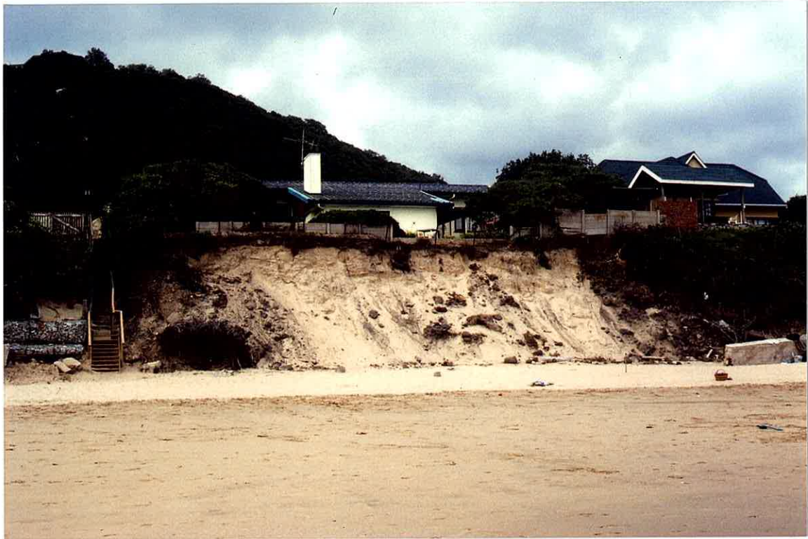
Photo 39. Here is more devastation where the long middle section of the retaining wall has just disappeared, leaving the rondavel dwelling above very close to plunging down the sand dune cliff.
