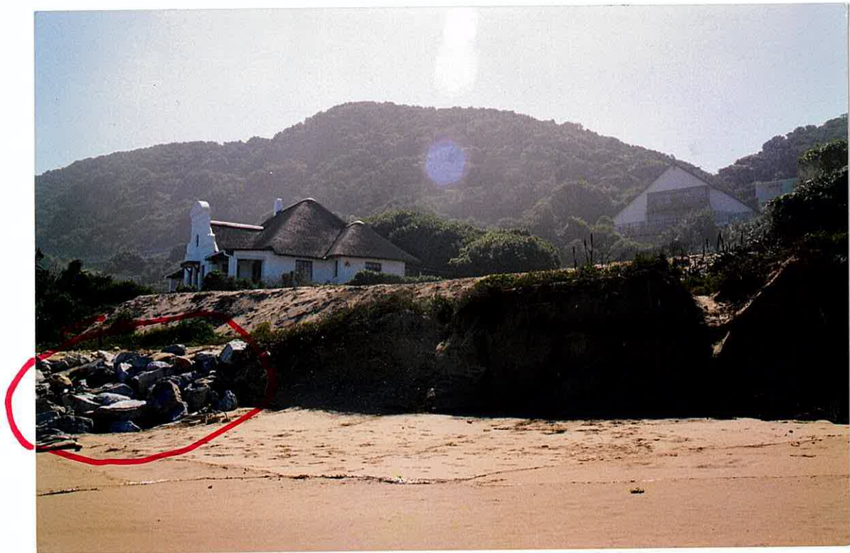
Photo 37. Here, moving Eastwards from where the neighbour's rock barrier (ringed in red) ends, the sand dune has now been reduced to an unstable sand cliff
