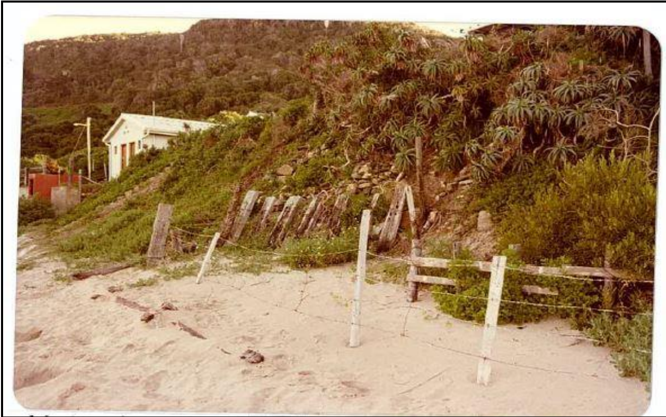
Figure 8: Front view of sand dune showing the top ridge of the low sloping dyke protruding from the sand dune.
