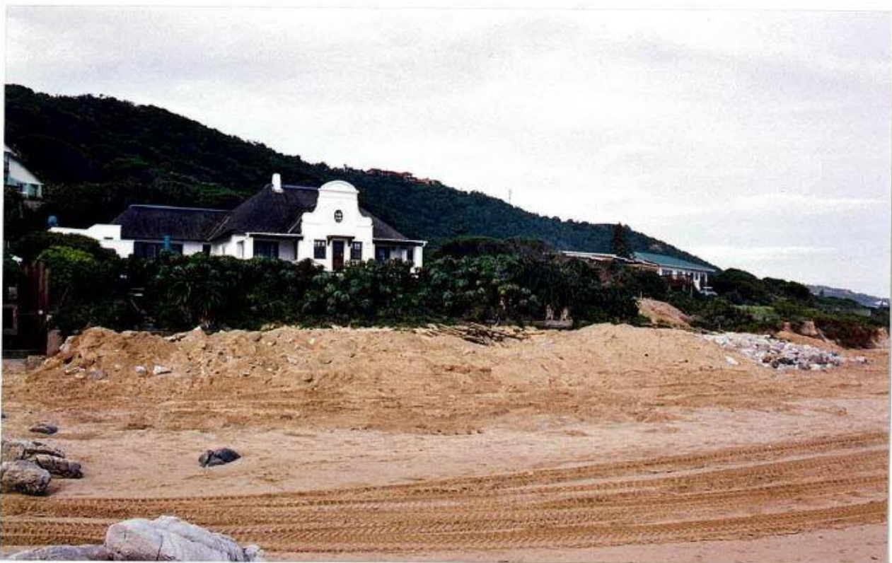
Figure 25: Completed rock revetment covered in a layer of beach sand.
