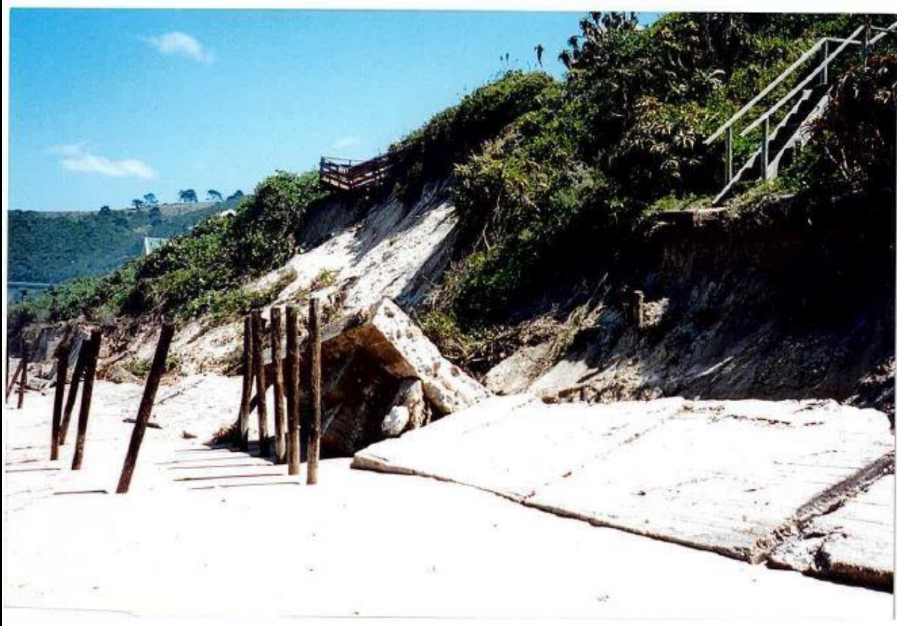
Figure 20: Damage to a retaining wall along the Wilderness Beach due to the above mentioned high tide event.
