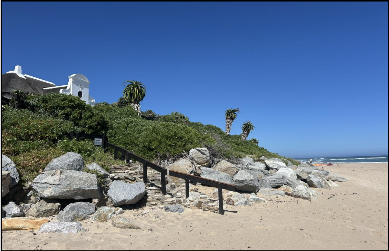
Figure 32: Rock revetment and beach access.
