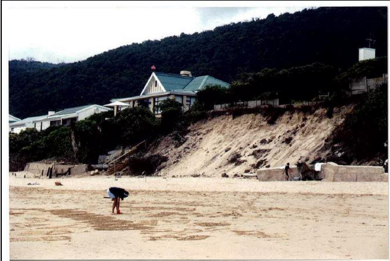
Figure 21: Damage to retaining wall and dune along Wilderness Beach due to the above mentioned high tide event.
