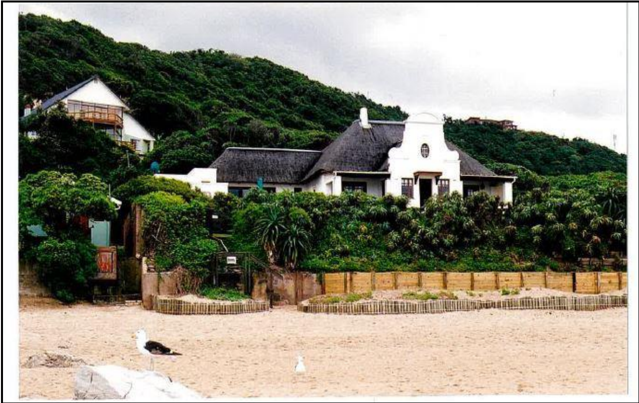
Figure 17: House with wooden gabion installed and beach access.
