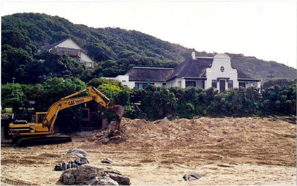
Figure 24: Front end loader placing the final few rocks in place and covering them with a layer of beach sand.
