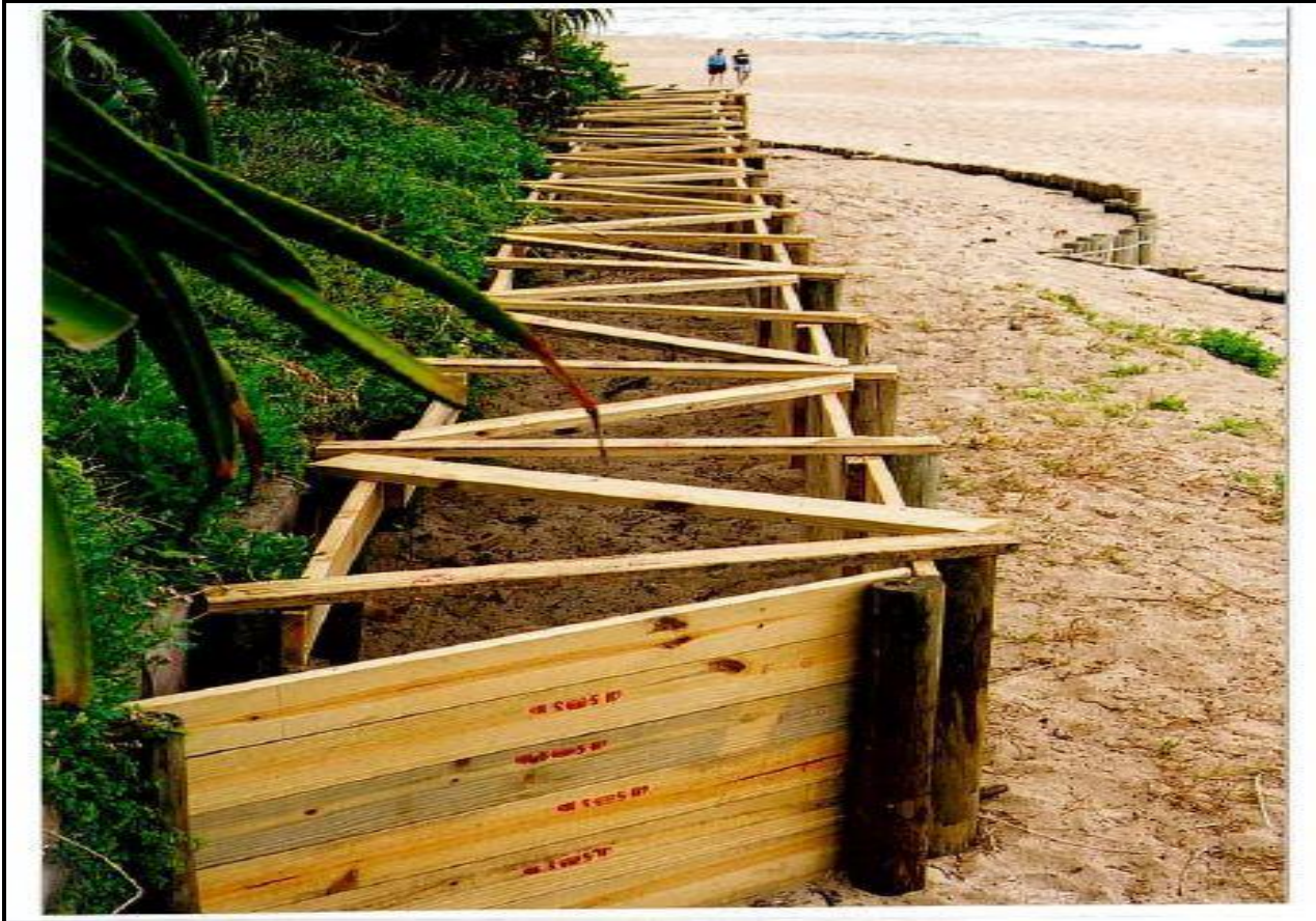
Figure 16: Wooden gabion being constructed.
