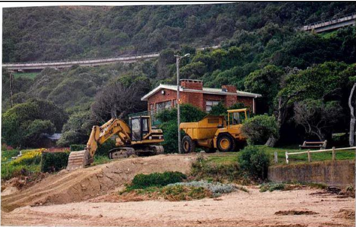
Figure 23: Access ramp for front end loader to gain access to the beach from the public picnic area.
