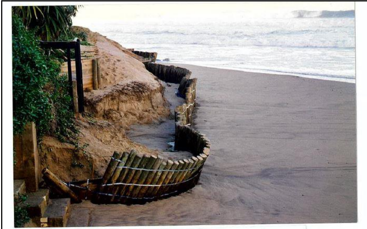
Figure 19: Damage to barrier poles.
