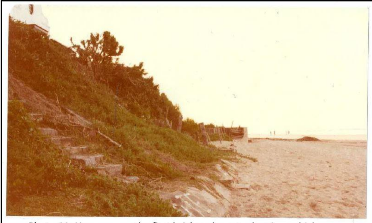
Figure 6: First brick mortar barriers installed at the property boundary at beach level. In the foreground is the low sloping dyke and beach access. Further along is the curved reinforced wall.
