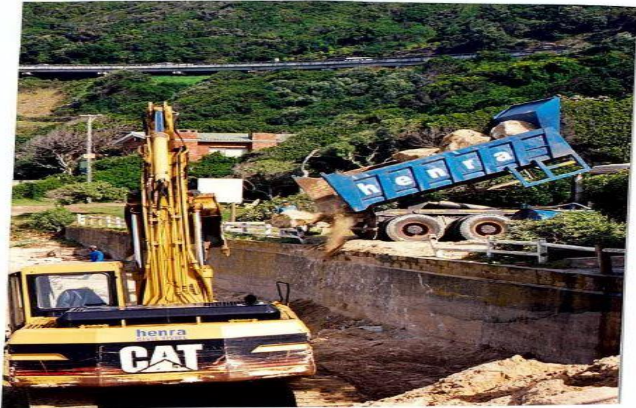
Figure 22: Rock boulders being tipped off onto the beach from the public car park.
