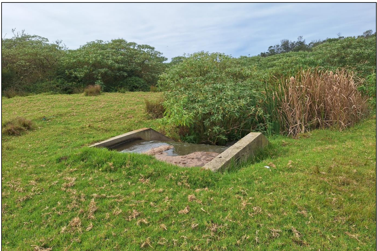
Plate 2: Photograph of the outlet structure discharging effluent into a channel towards the wetland
