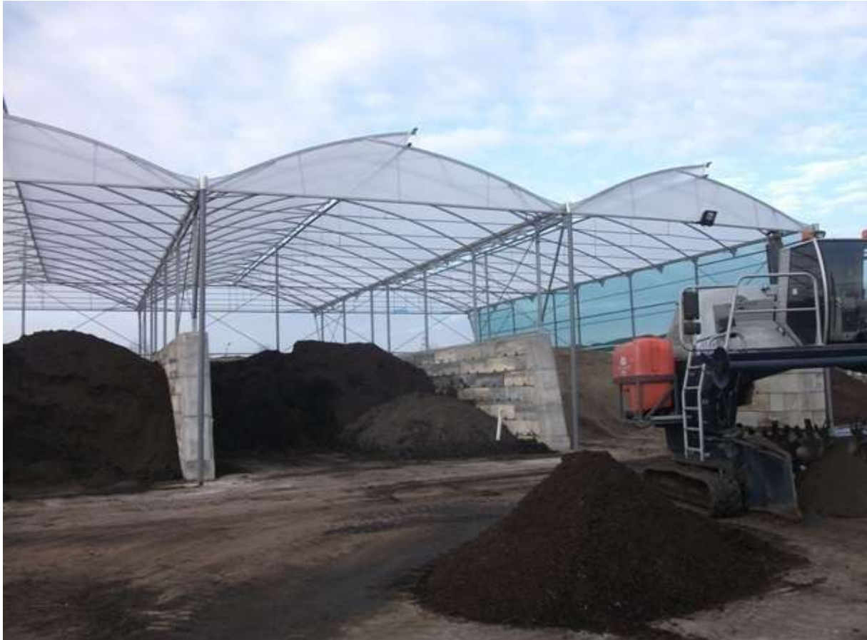
Figure 6-15: An Example of sludge storage bunds with concrete floors and translucent roof covers.
