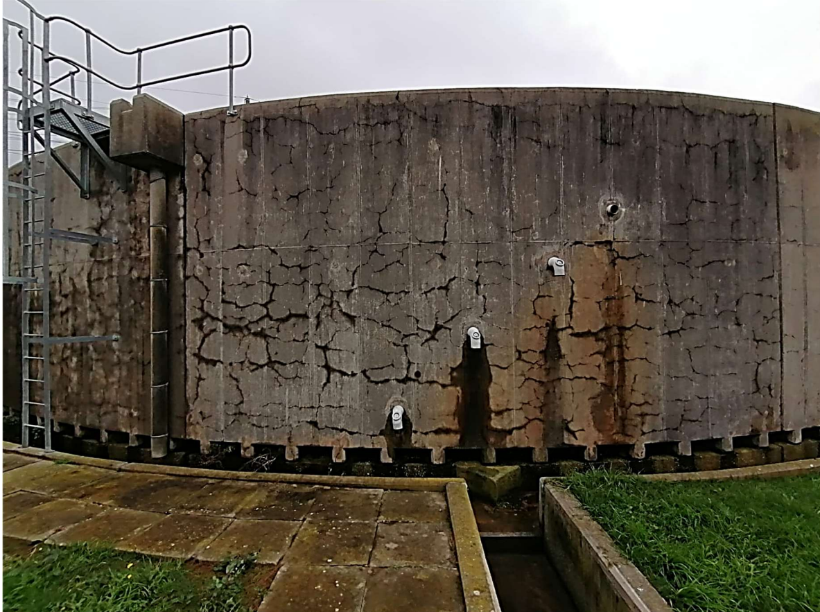
Figure 4-3: Cracks visible in bio-trickling filter walls
