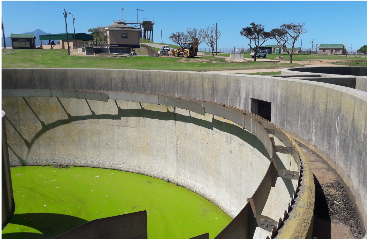
Figure 4-4: Inside of Existing PST
