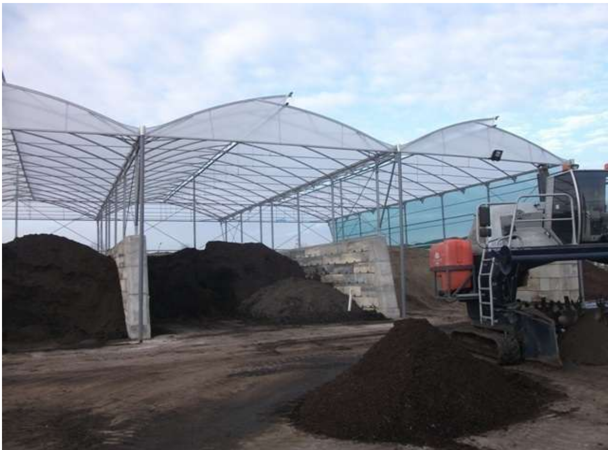
Figure 7-29: An Example of sludge storage bunds with concrete floors and translucent roof covers.
