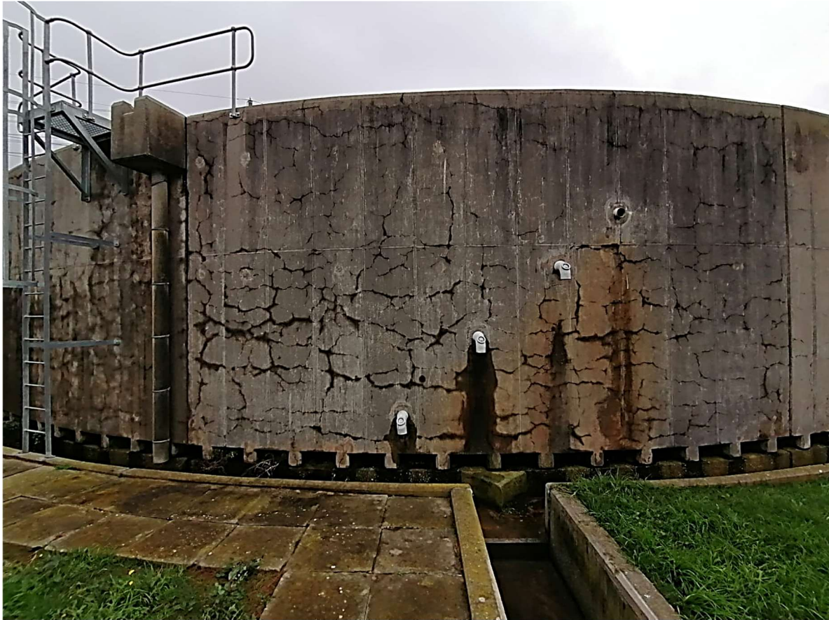
Figure 4-3: Cracks visible in bio-trickling filter walls
