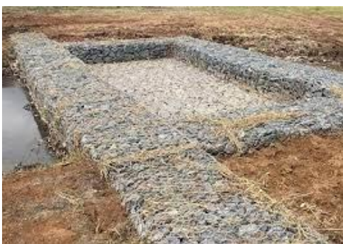
Figure 24 & 25 – Accepted general outflow structure erosion protection systems that are implemented in practice.
