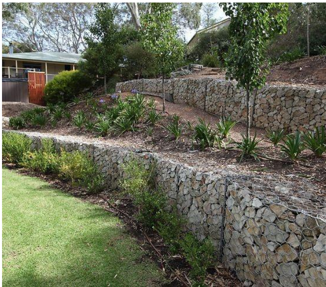
Figure 18 – Rock filled Gabion baskets in areas where retaining walls must be created.
