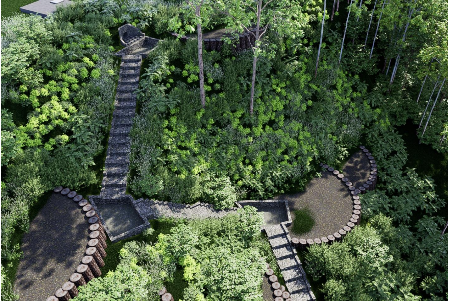
Figure 19 – Outflow Headwall structure into 1 st stilling pond, followed by 1 st water stair section to the 2 nd stilling pond.
