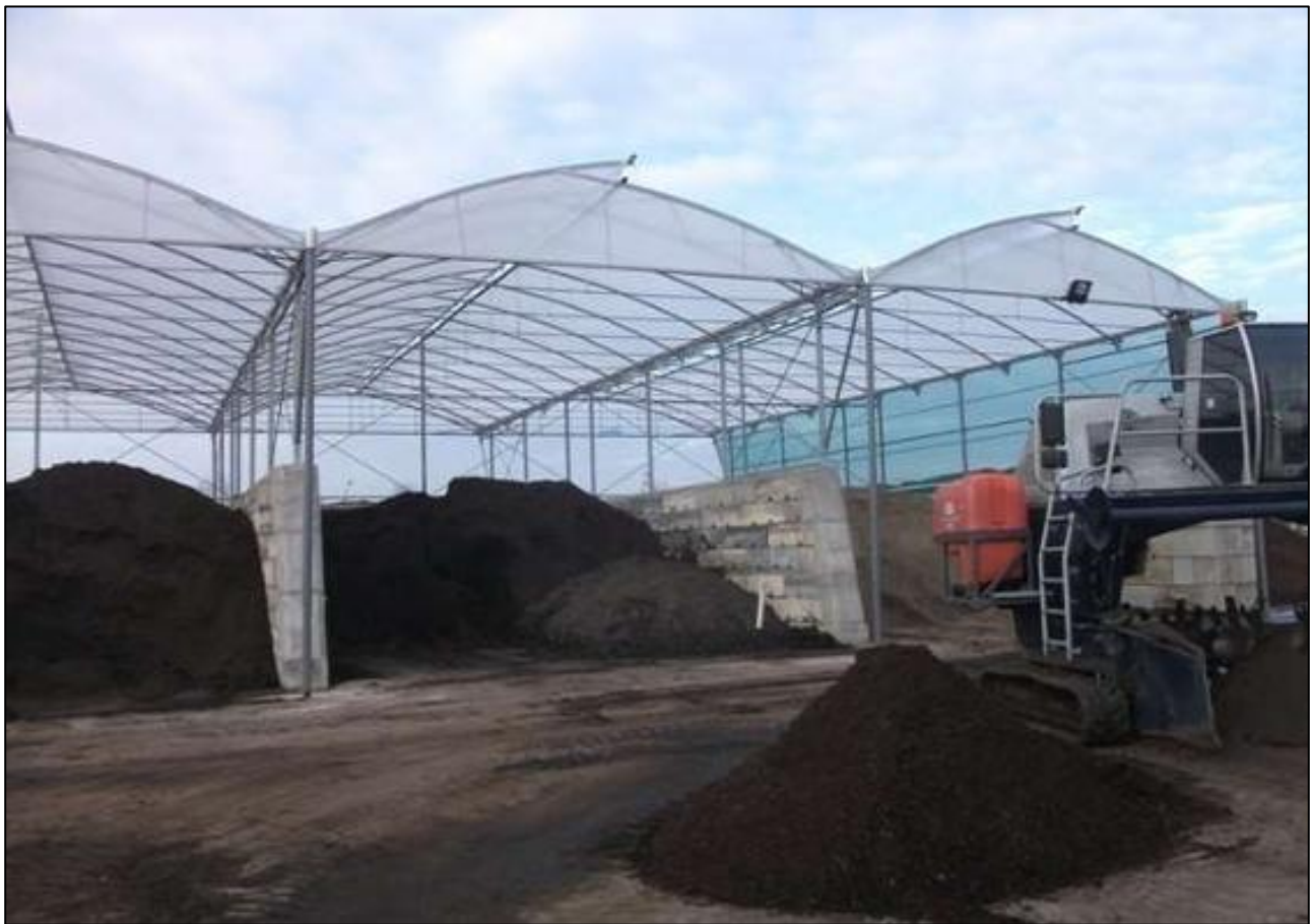
Figure 10: An Example of sludge storage bunds with concrete floors and translucent roof covers.
