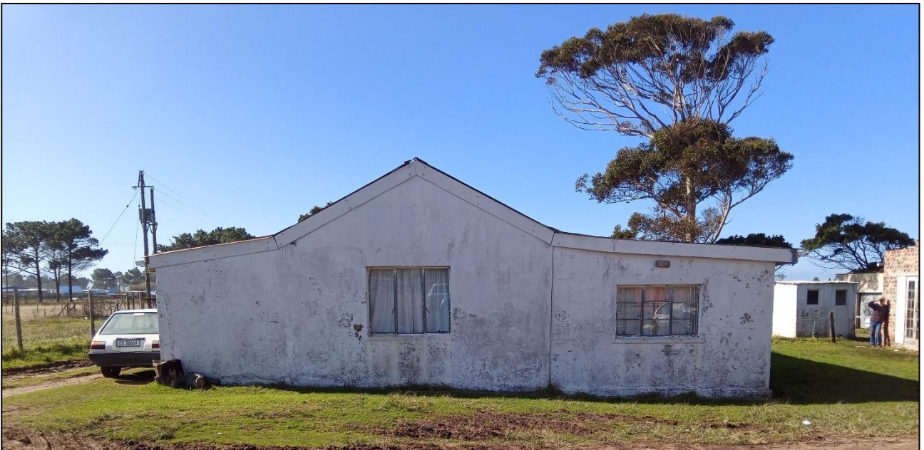
West end of historical cottage in the northeastern part of Portion 7 showing that the southern lean-to was added later.
