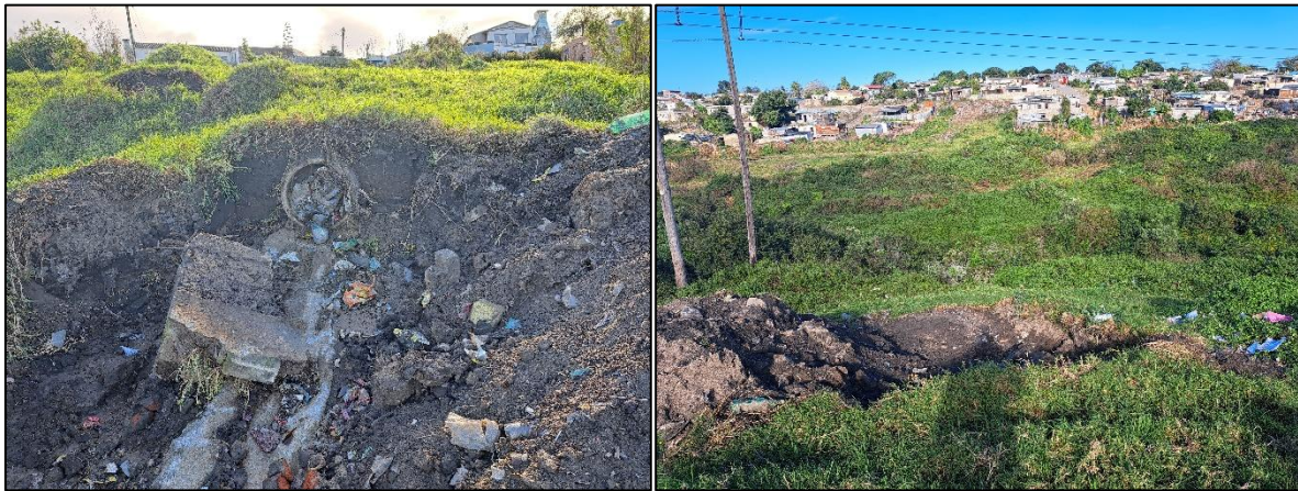
Figure 16: Photographs of RSW5 showing the blocked outlet pipe, demolished headwall and excavation.
