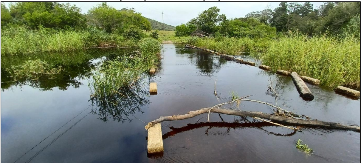
Plate 3: A photograph taken of the old road crossing the Moordkuil River, which acts as a weir for the pumpstation
