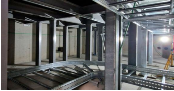
Figure 4-12: False floor example typically used in data centres
