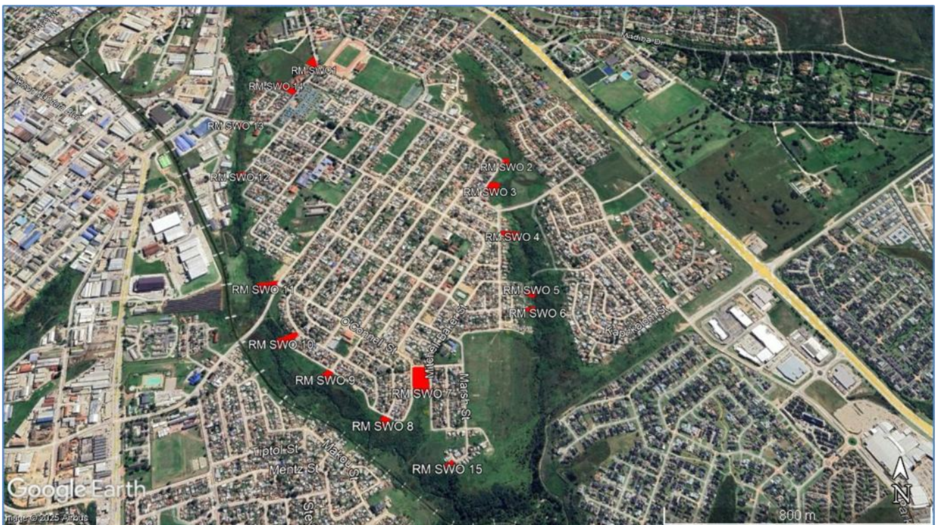
Figure 3: Stormwater Outlets structures (1-15).
