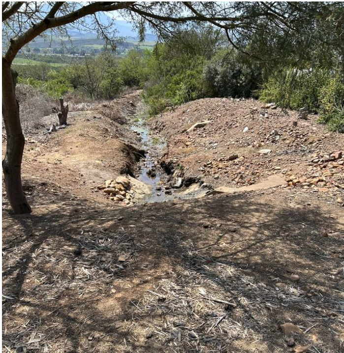
FIGURE 4: EXISTING STORMWATER CHANNEL ADJACENT TO ERICA STREET INTO WHICH THE SITE RUNOFF WILL BE DISCHARGED
