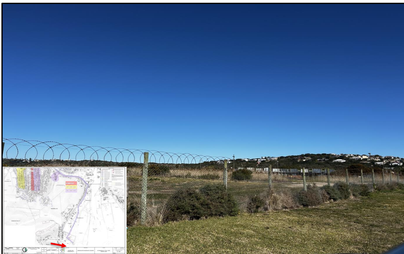
Figure 10: Southern section of pipeline route.
