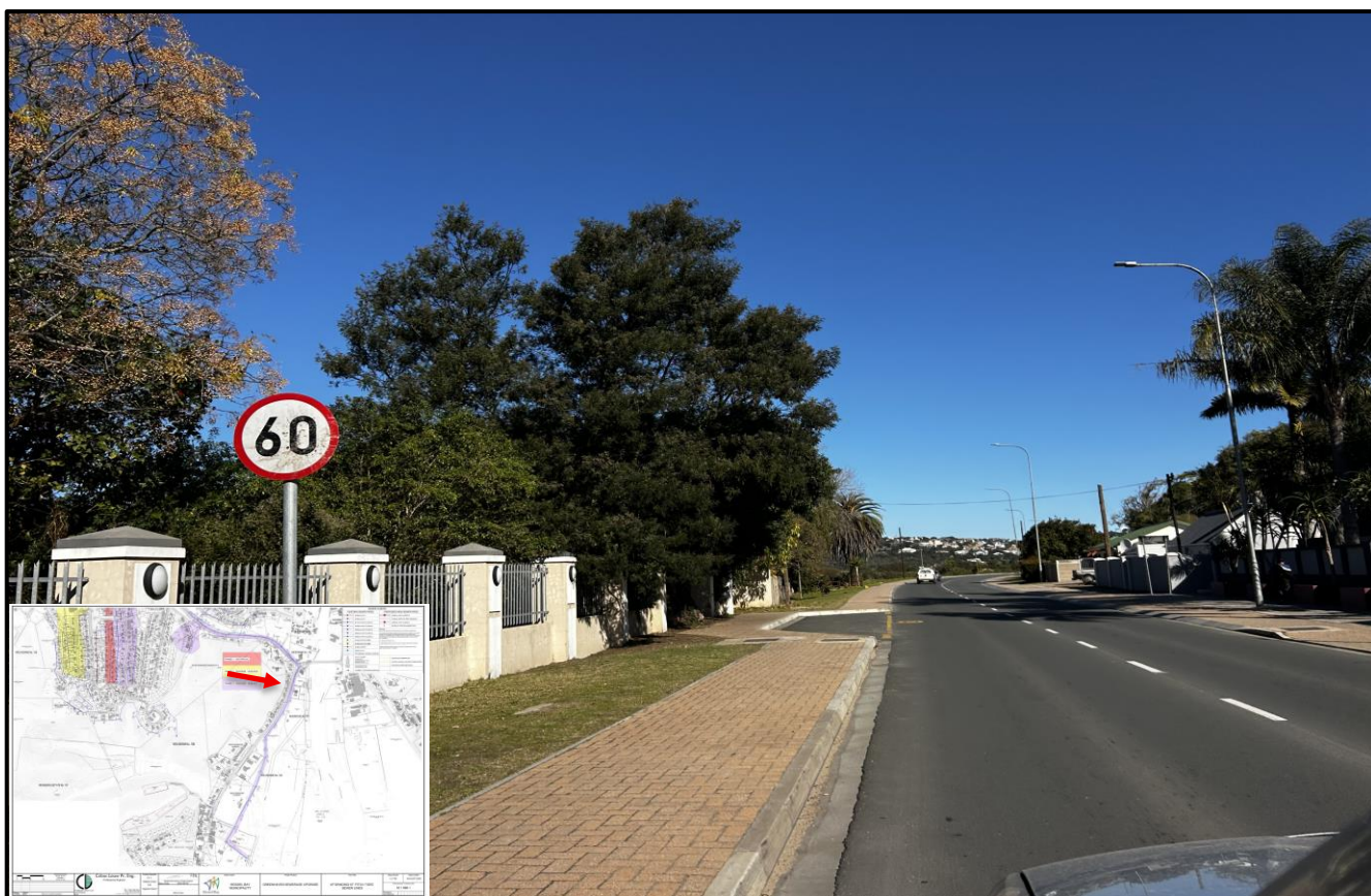
Figure 2: Section of pipeline heading down Long Street from the traffic circle towards the south.
