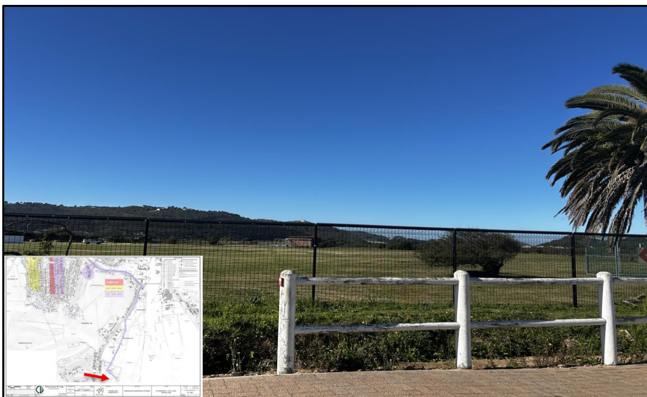
Figure 11: Southern end of pipeline route at the cricket field sewerage pump station.
