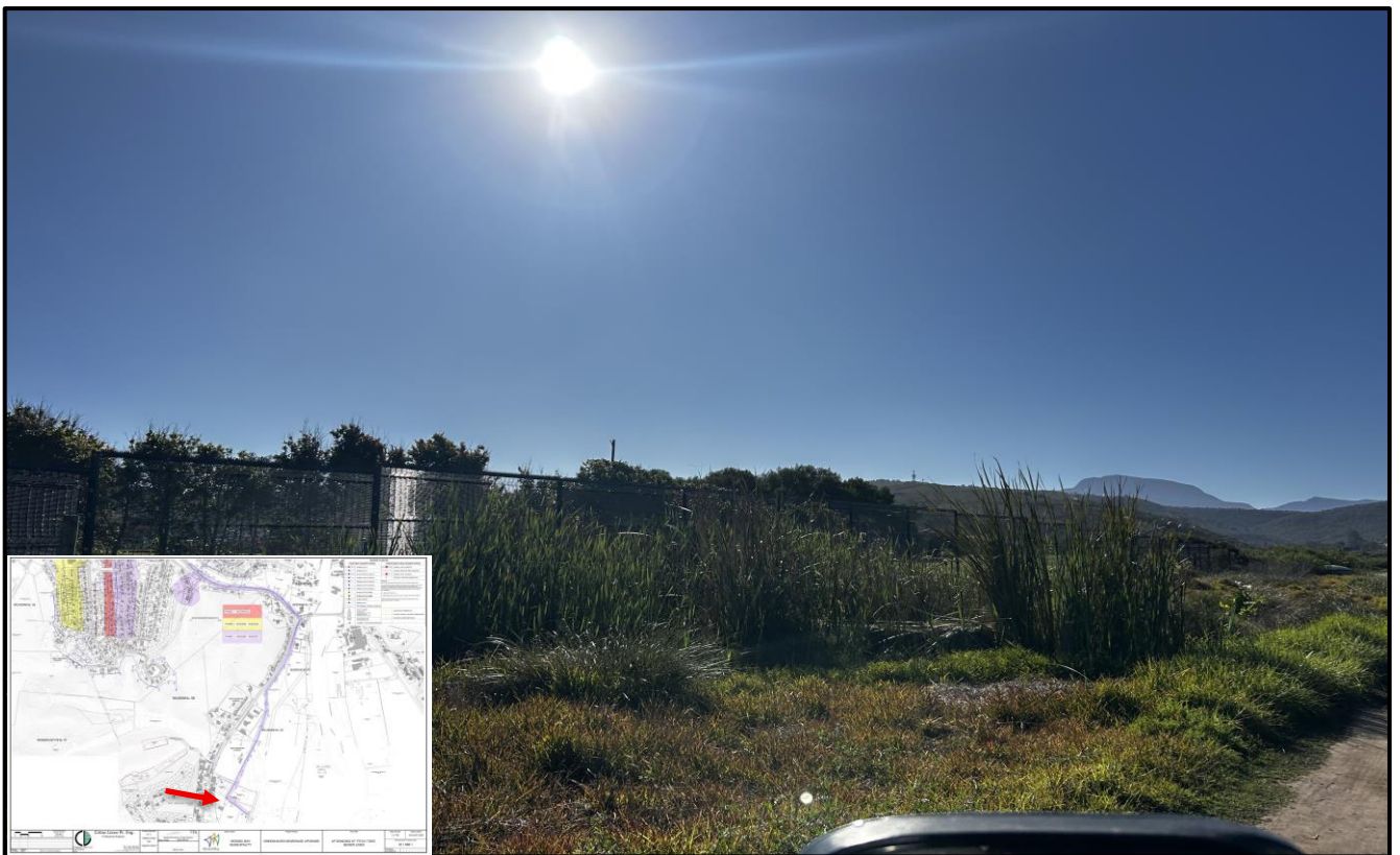
Figure 9: Lower southern section of pipeline route.
