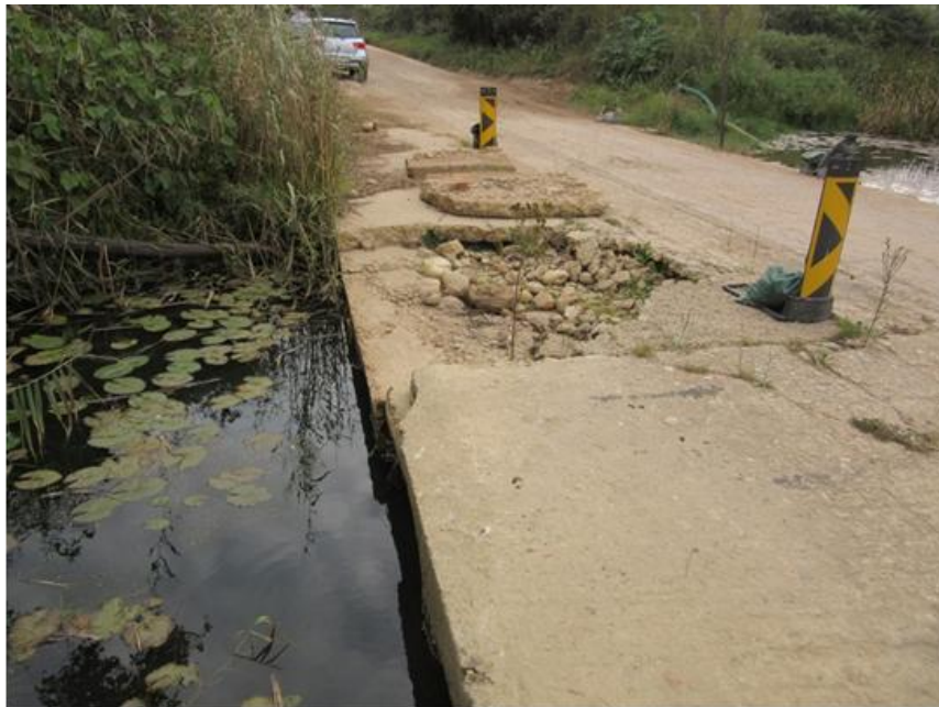
Figure 4: The upstream side of the causeway
