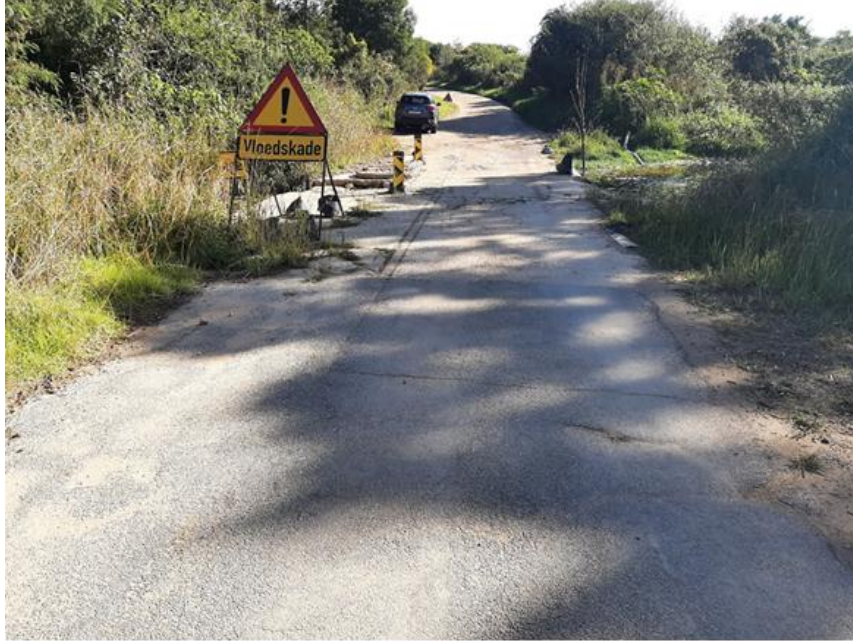
Figure 1: A view of the road and causeway from East to West
