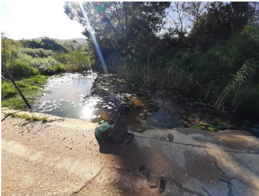
Figure 3: The downstream side of the causeway
