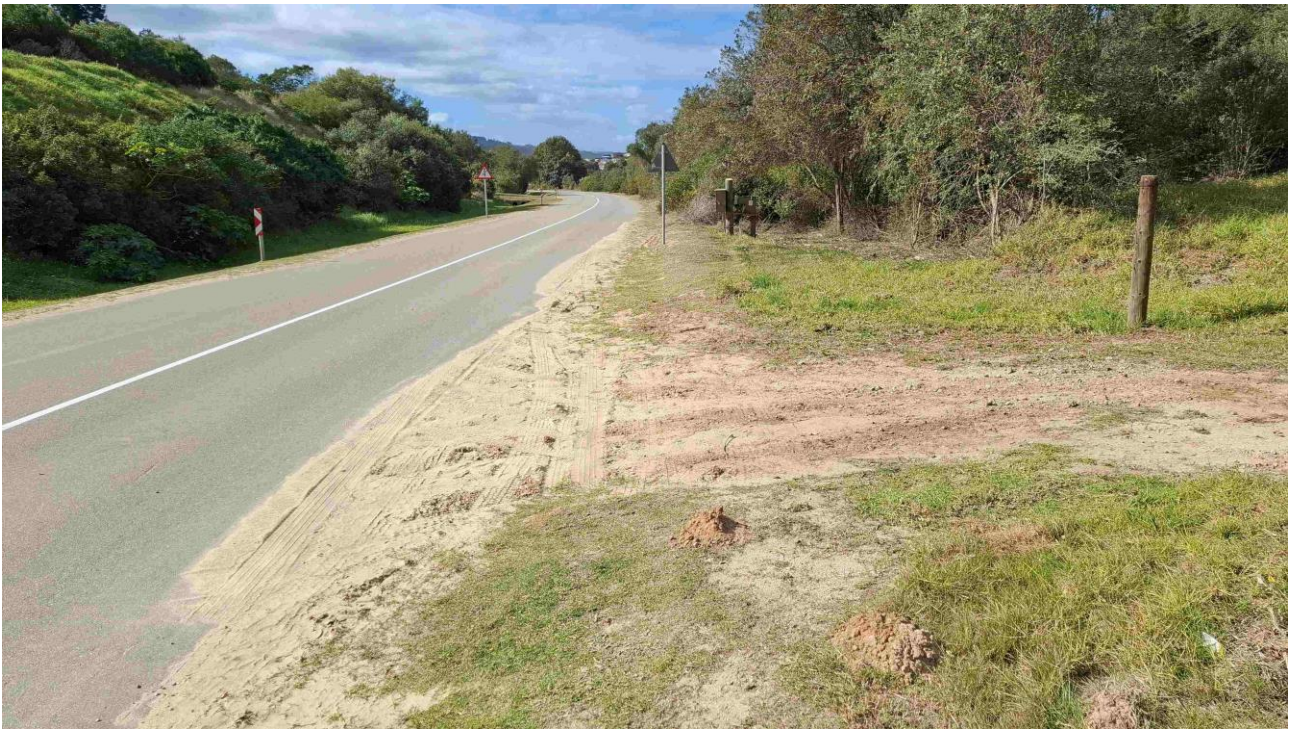
Figure 3. Typical site conditions of the assessed area.
