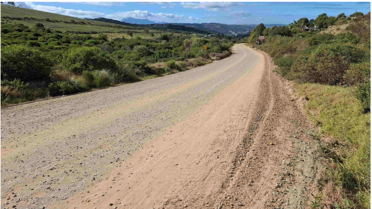
Figure 4. Typical site conditions of the assessed area.
