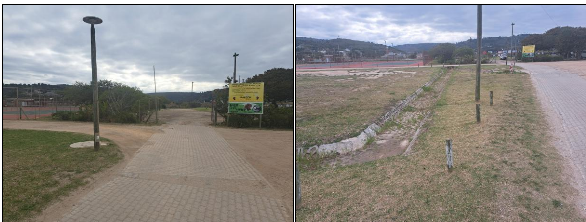
Figure 11: Paved roads and sports fields in Zone E (left and right).
