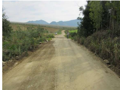
Road DR1639 at km 1.63; upstream on RHS.
