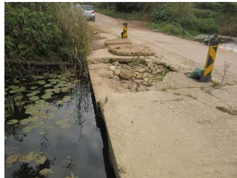
Water ponding upstream of drift. Damage to deck caused during previous flood.
