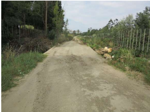
Road DR1639 at km 1.63; upstream on LHS.
