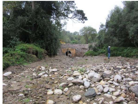
Downstream – looking towards culvert
