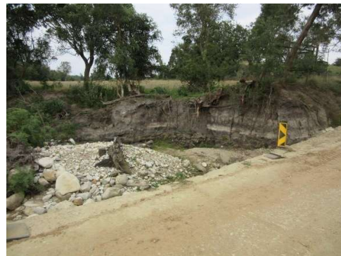
Downstream – looking away from culvert
