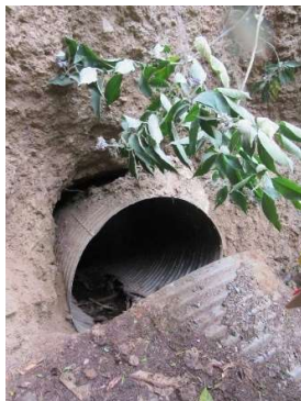
Downstream section of the Armco culvert washed away and collapsed due to erosion
