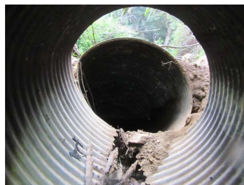
Downstream section of the Armco culvert washed away and collapsed due to erosion
