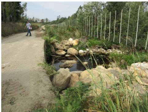
Rip rap has recently been placed on the downstream side to reduce scour
