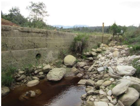
Downstream – looking towards culvert
