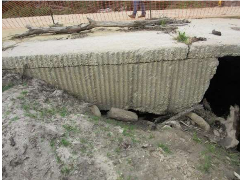
Upstream – looking towards culvert
