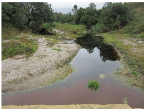
Upstream – looking away from culvert
