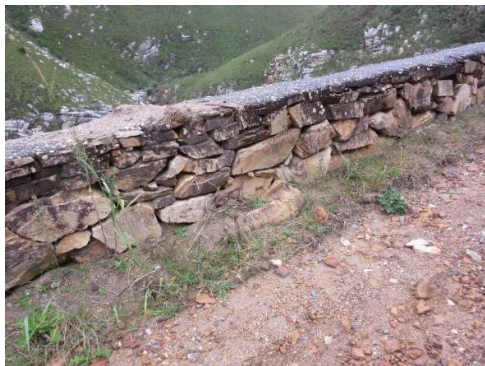
Image of existing dry-stack balustrade wall in Montagu Pass on road DR1640
