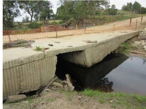
Upstream – looking towards culvert
