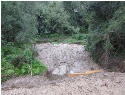
Downstream – looking away from culvert
