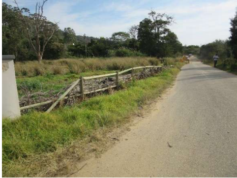
Road DR1791 at km 1.59; upstream on LHS. Debris from previous flood trapped against fence.
