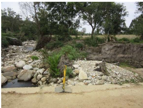
Downstream – looking away from culvert
