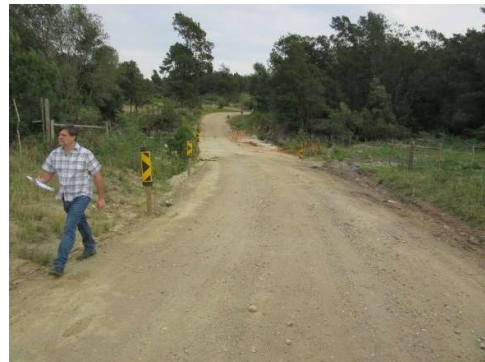
Road DR01633 at km 3.35; upstream on RHS.
