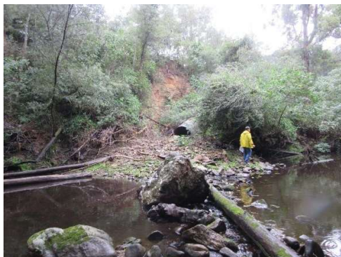
Downstream – looking towards culvert
