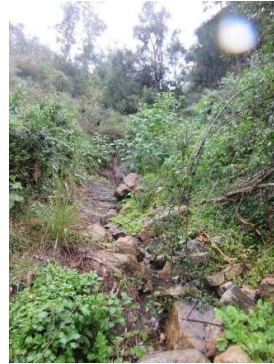
Upstream – looking away from culvert
