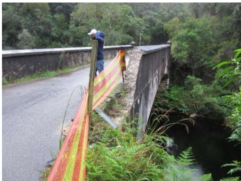
One of the end-blocks and part of the balustrade to the Salt River bridge on road MR00355 at km 8.67 was knocked down by vehicle impact. This is on the RHS when approaching the bridge from Saasveld side.
