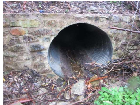
Head fall and culvert inlet
