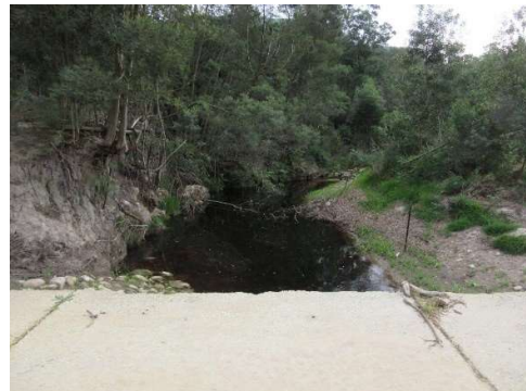
Upstream – looking away from culvert
