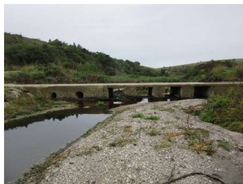
Upstream – looking towards culvert
