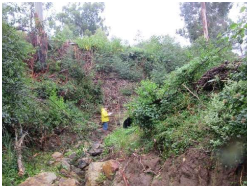
Upstream – looking towards culvert
