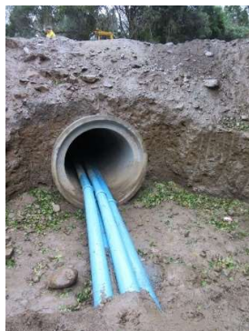
Upstream – looking towards culvert
