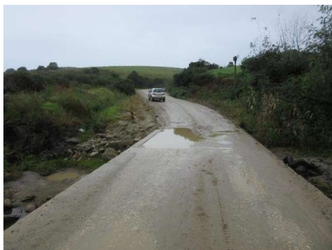
Road DR1602 at km 8.48; upstream on RHS.
