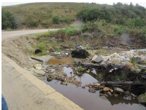
Downstream – looking away from culvert
