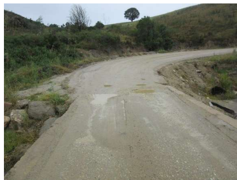
Road DR1602 at km 8.48; upstream on LHS.
