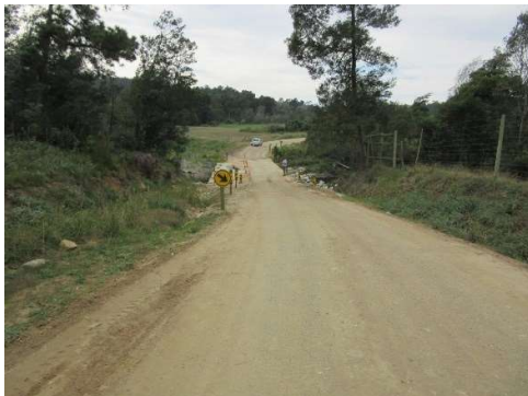
Road DR01633 at km 3.35; upstream on LHS.
