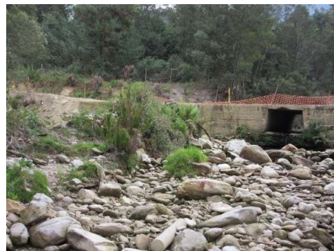
Downstream – looking towards culvert
