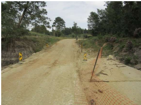
Road DR01633 at km 3.35; upstream on RHS.
