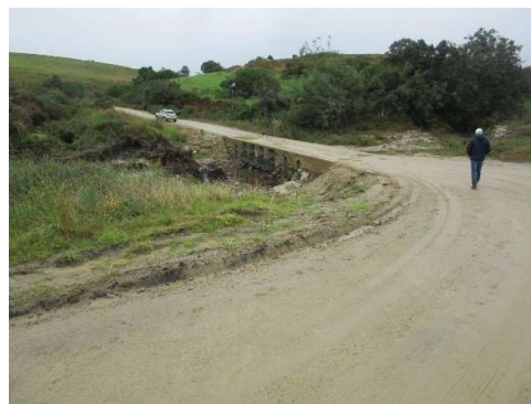
During the November 2021 flood the George side approach road was washed away for a length of 15m. This portion of road has been repaired and widened
