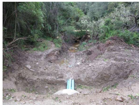
Upstream – looking away from culvert
