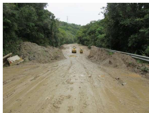
Road MR00355 at km 3.77; upstream on LHS. Backfilling in progress.
