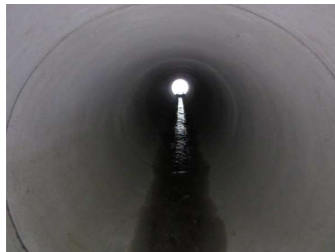
Inside newly installed pipe culvert
