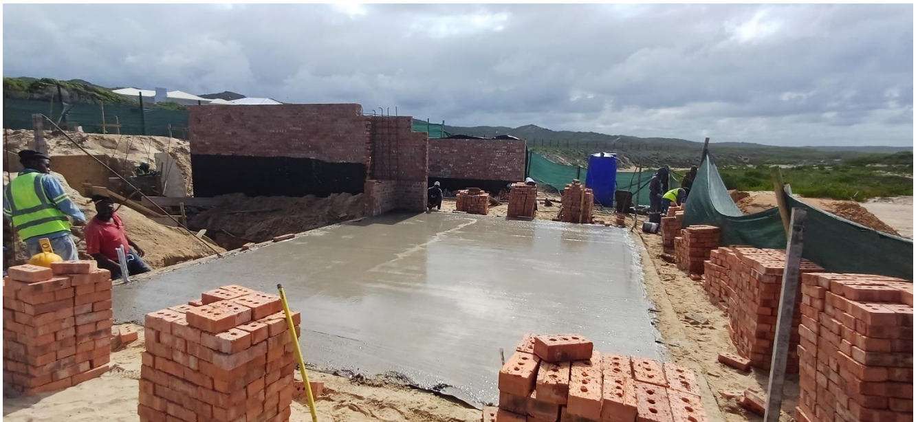
Photo 4: Ready-mixed concrete was used to cast the floor of the double garage on Erf 2457. Note the retaining walls of the main house in the background. The cavity in these walls will also be filled with ready-mixed concrete.
