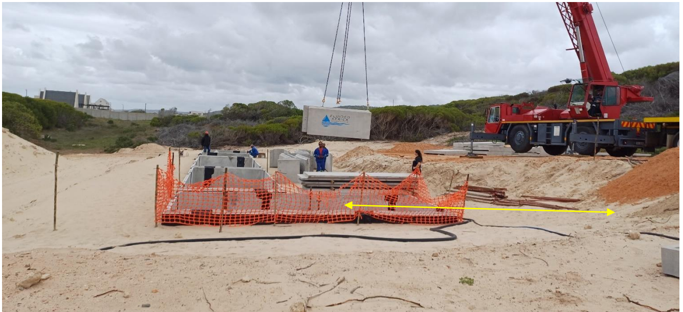
Photo 6: The last of the pre-cast concrete panels were off-loaded on site on 13 March 2024. These panels will form the last row of panels to be placed on top of the package sewage plant. The crane was off-loaded from a low-bed truck with a full tank of diesel.
