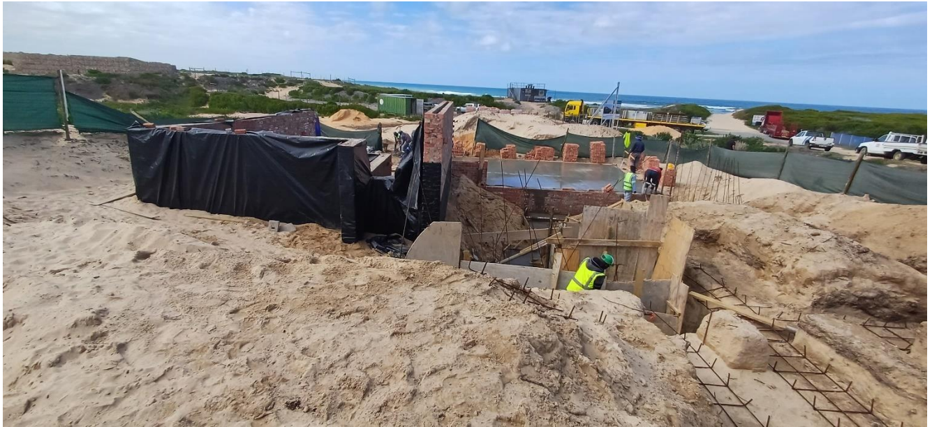
Photo 7: Shutter boards were required to hold back sand from falling into deeply excavated foundations for the house on Erf 2457.
