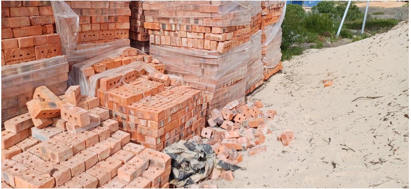
Photo 1: The building materials on the site of the first house are stored in a non-sensitive area, and in a neat condition. The building site supervisor was reminded to store plastic wrapping and used cement bags in a lidded bin for later removal from site.
