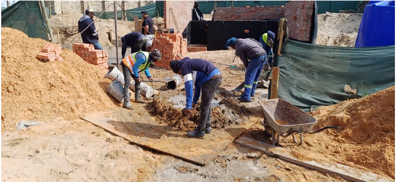
Photo 5: Mortar is being mixed on mortar boards on site for the building of walls and retaining walls.
