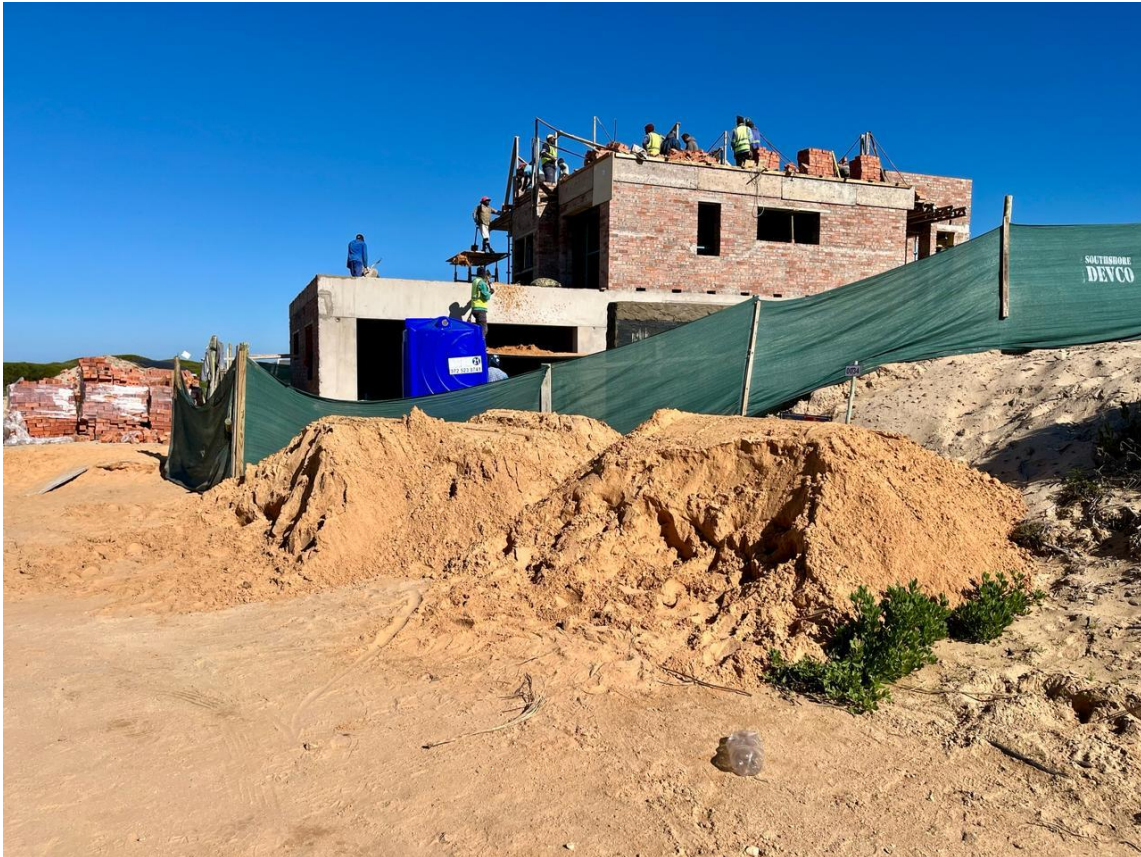
Photo 3: The building materials are neatly stored on site of the house on Erf 33.
