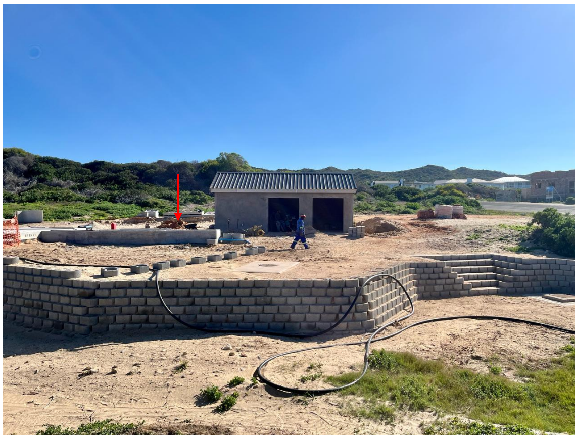
Photo 1: The building materials on the site of the sewage package plant are stored in a non-sensitive area, and in a neat condition. Some builder's rubble is being generated (red arrow) and must be removed from site on a weekly basis or put into a skip. The sewage works control room is nearing completion.
