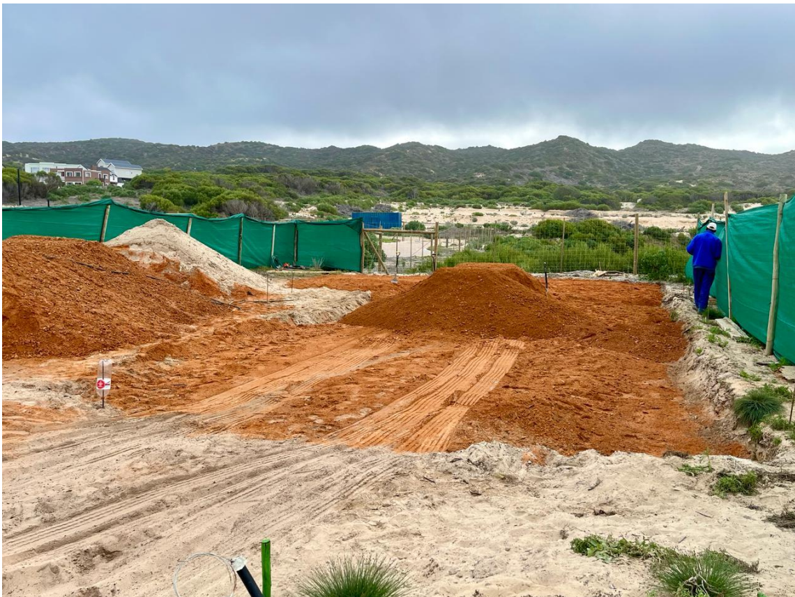
Photo 4: Construction work has started on Stand 44/Erf 2382 by Southshore Devco, with the excavation of sand from the building platform. G7 material is being placed within the excavated building platform, which will be compacted, for creating a stabilized raft foundation. The shade cloth is being erected on the boundary of the erf.
