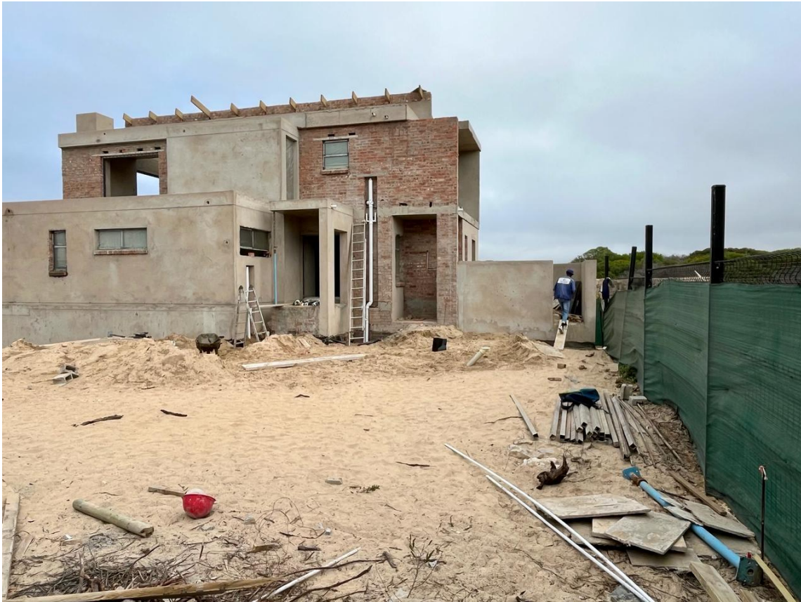
Photo 3: The roof is being constructed. Shutter boards and scaffolding are neatly packed on the inside of the erf.
