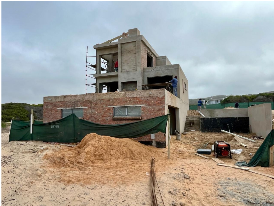
Photo 2: The main construction of house on Stand 33/Erf 2457 is nearing completion. Some outside walls still need to be plastered and clad with natural limestone blocks.
