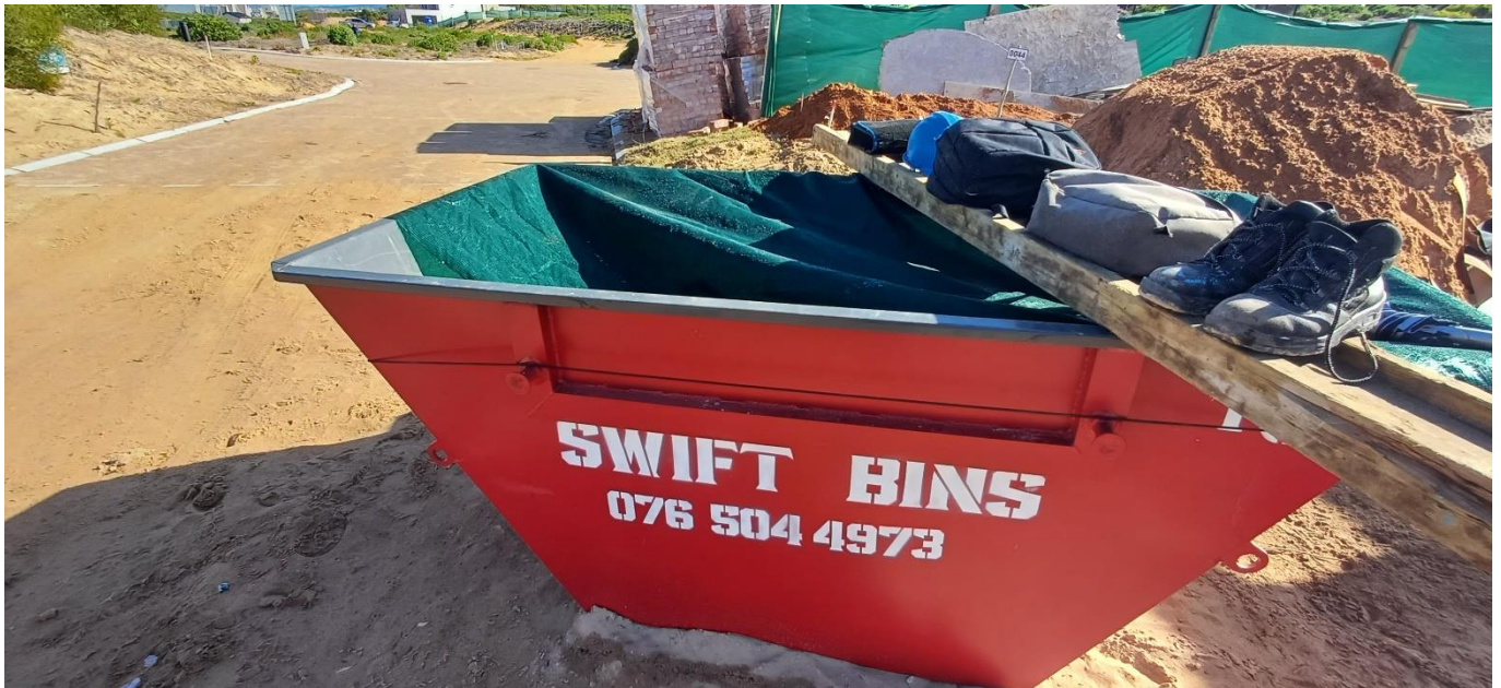
Photo 3: Dedicated waste skips are being used to contain builder's rubble and general waste. Shade netting is used to prevent litter from being blown around the site.
