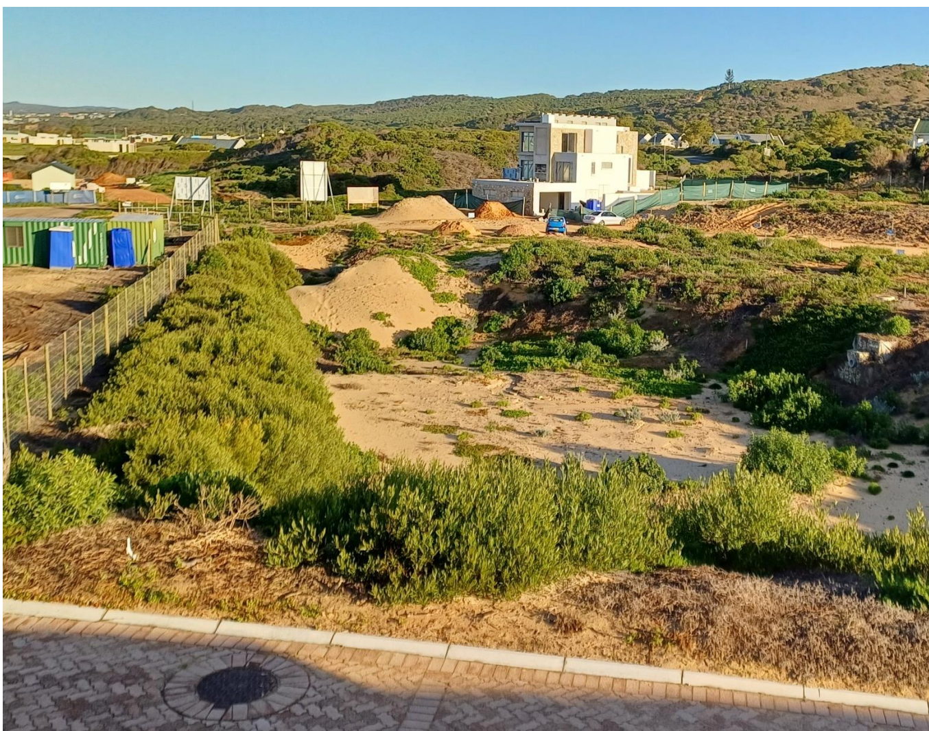
Photo 2: The construction of house on Stand 33/Erf 2457 is nearing completion. The outside walls are being painted and the tiling of the decks and floors inside the house is being undertaken.
