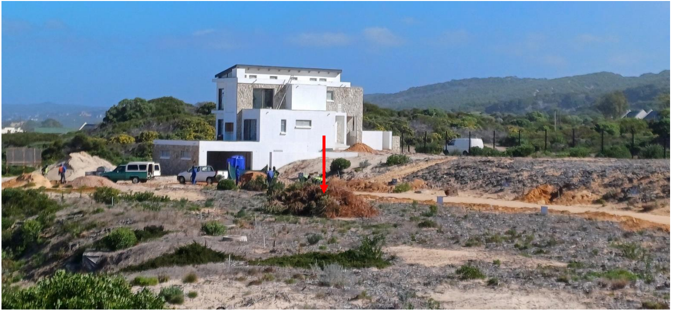
Photo 3: The construction of house on Stand 33/Erf 2457 is nearing completion. The roof is on and the outside walls have been painted. The tiling of the decks and floors inside the house have been completed and the inside fittings are currently being fitted. Note the pile of alien vegetation that has been removed from the stands (red arrow).
