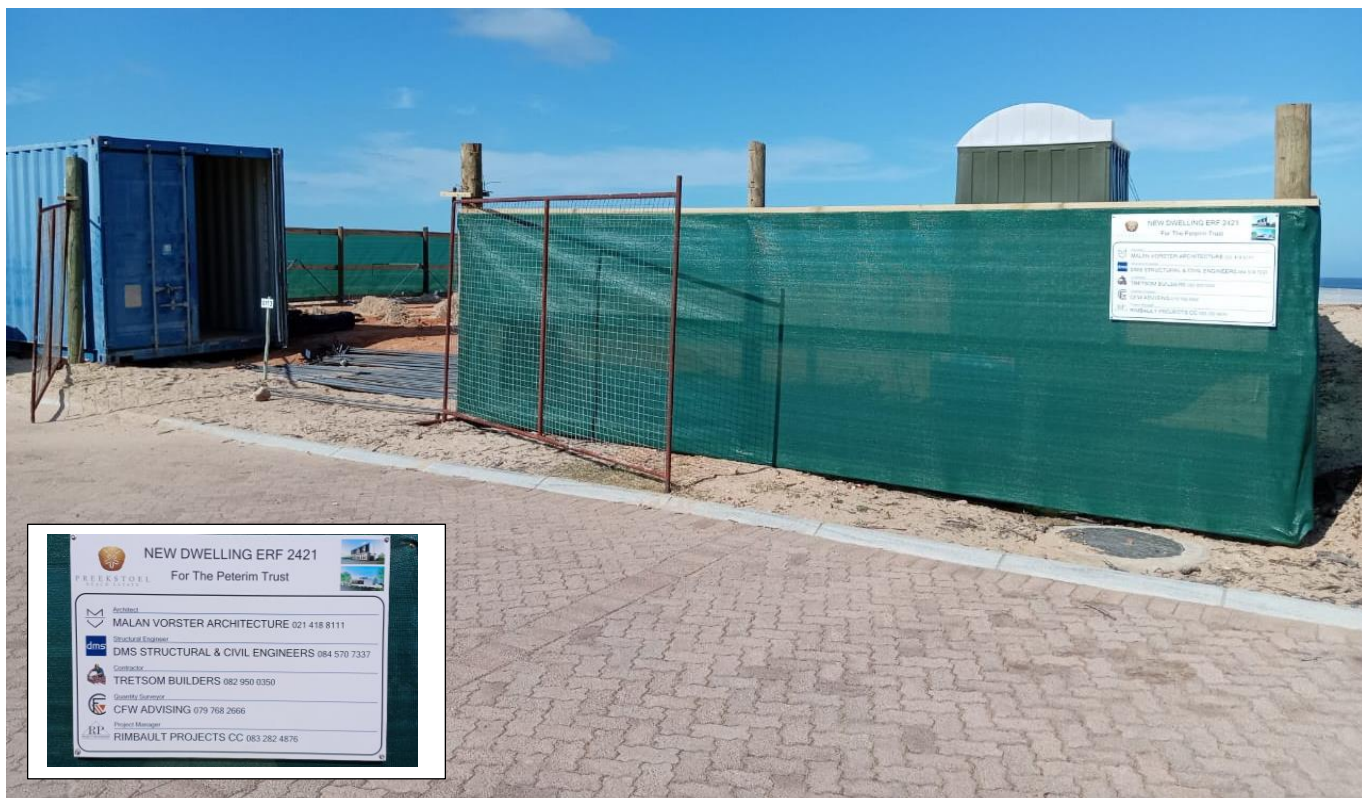
Photo 1: Construction of Stand 113 by Tretcom Builders has just started. Their notice board is on the perimeter shade cloth fencing.
