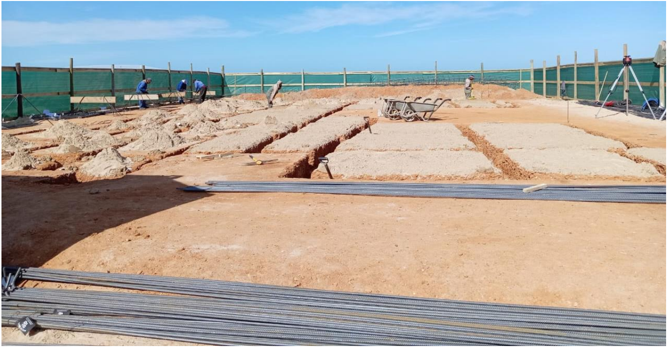
Photo 5: The G7 gravel layer has been compacted to its correct density and trenches have been excavated for the concrete beams. The staff in the top left corner of the photo are currently fixing the reinforcing “cages” for the concrete beams of the raft foundation of the house on Stand 113. The site has been neatly cordoned off with shade netting.
