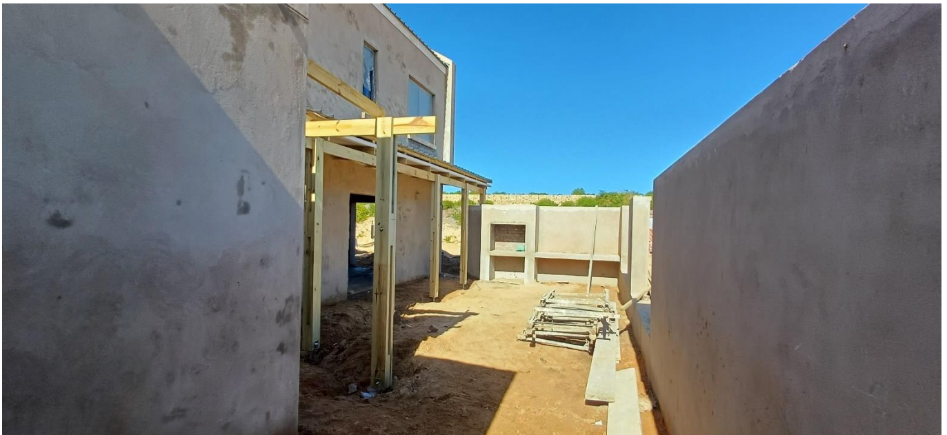
Photo 4: The wetwork of the house on Stand 44 has been completed.
