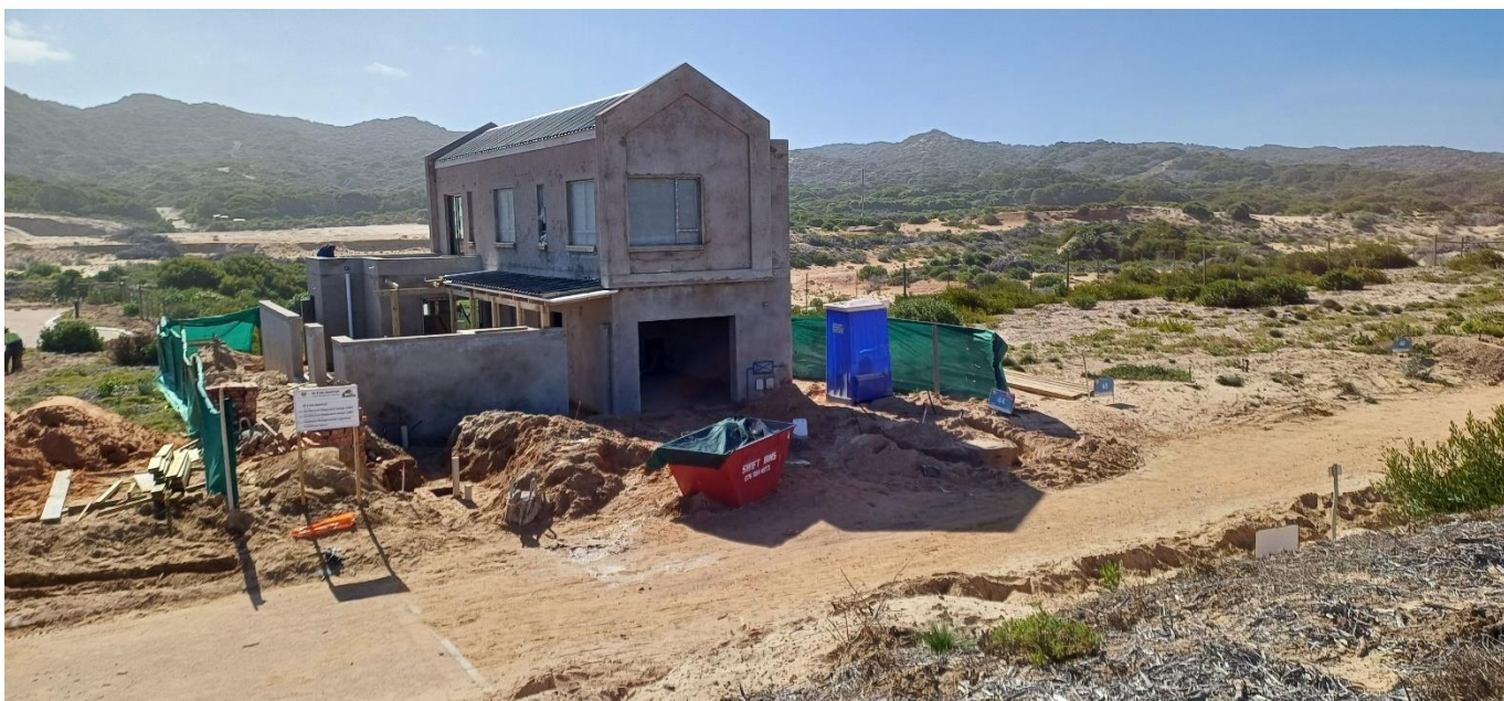
Photo 2: A waste skip is being used for the temporary storage of builder's rubble and general waste on Stand 44. The wet work has been completed for all intent and purpose and the roof is on.
